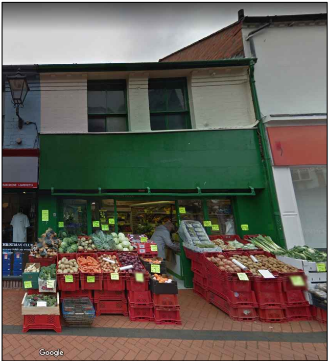
Historical Photograph 2 Henblas Street
