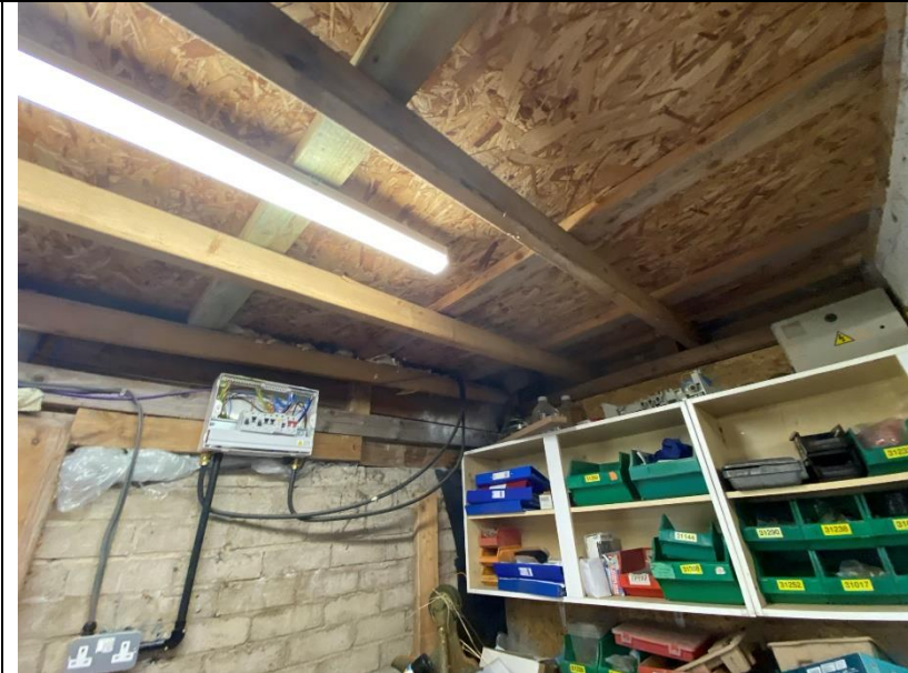
Interior of B3 (pictured above).
