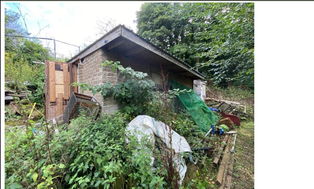
Northern and western elevation of B3 (pictured above).
