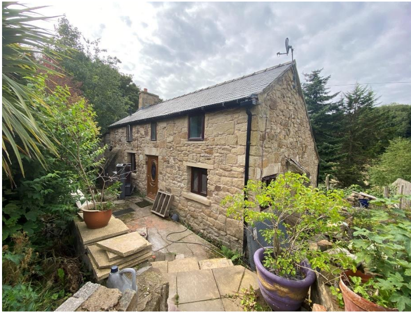
Eastern elevation of B1 (pictured above).
