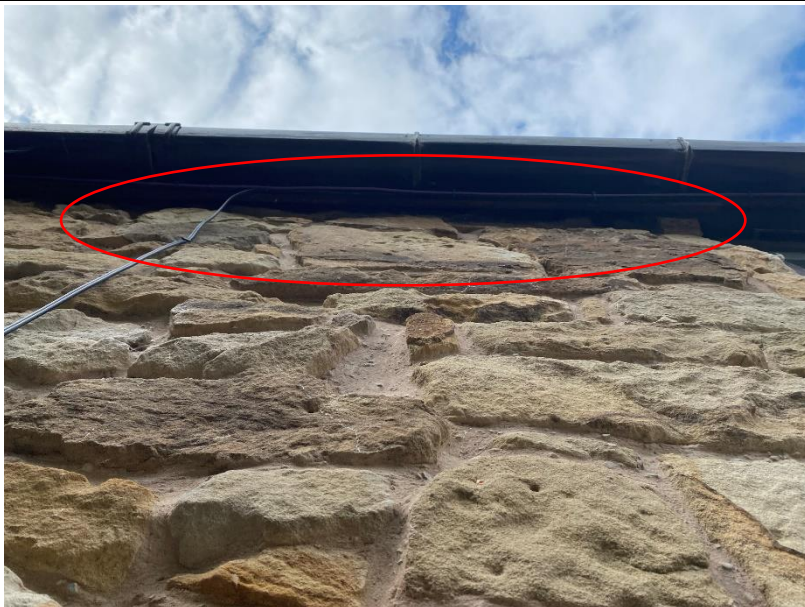
Eastern elevation of B1 (pictured above).
