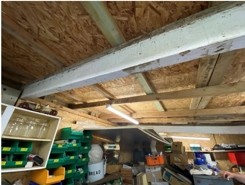
Interior of B3 (pictured above).
