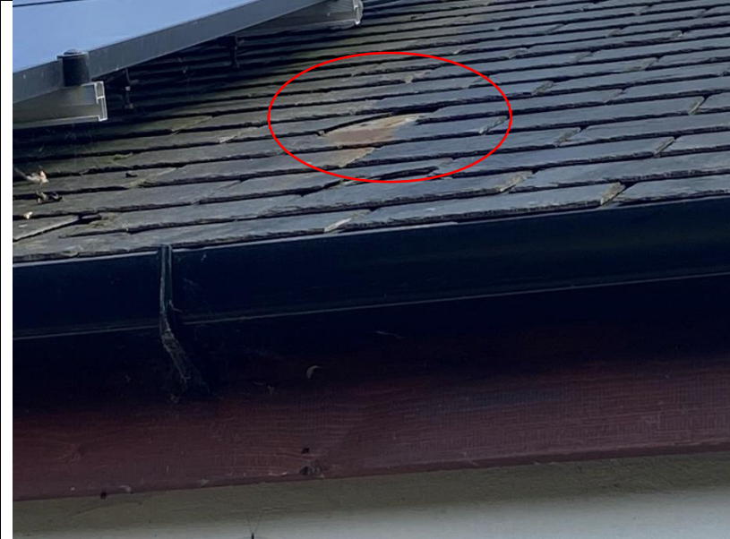
Western elevation of B1 (pictured above).
