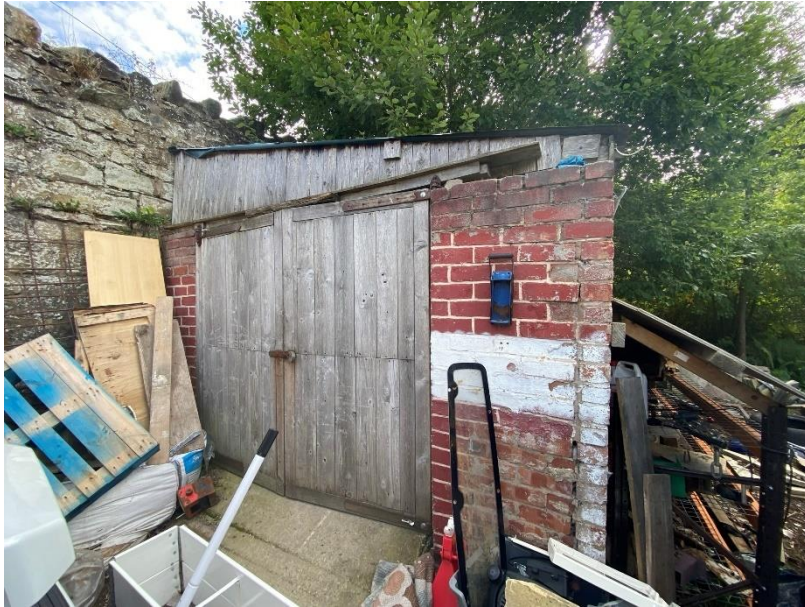
Northern elevation of B2 (pictured above).
