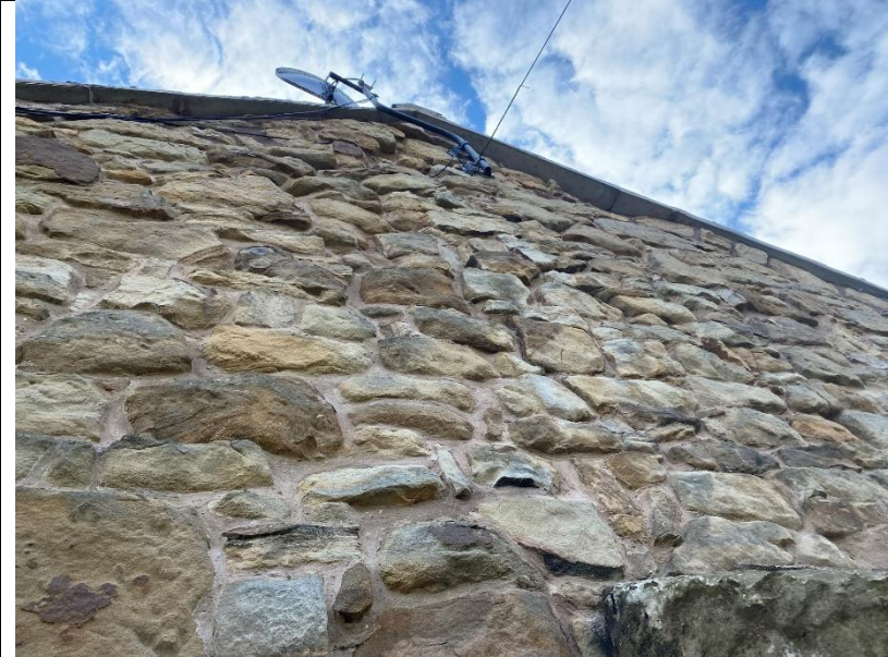
Northern elevation of B1 (pictured above).
