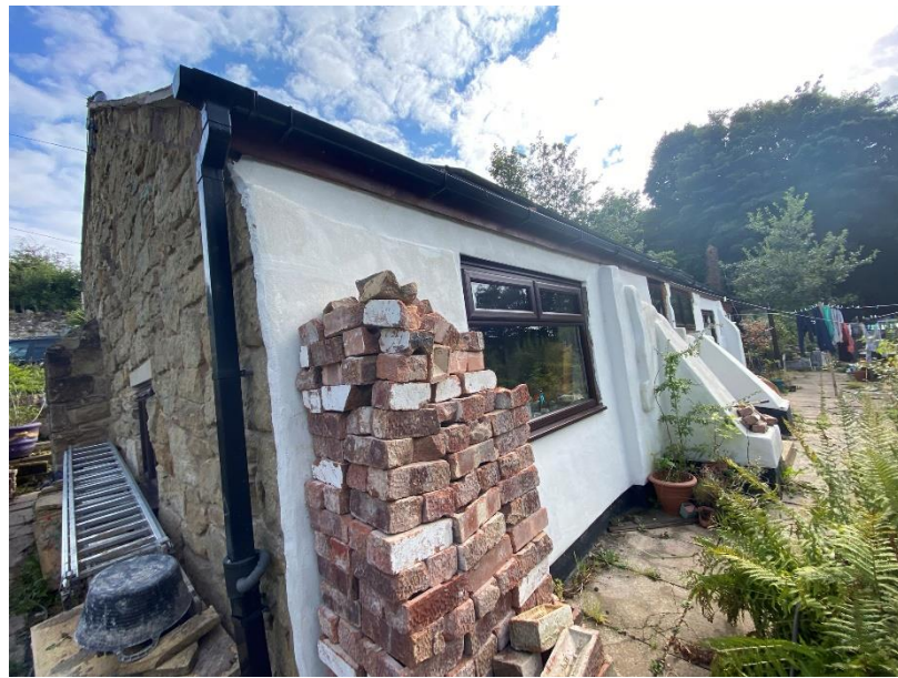
Western elevation of B1 (pictured above).
