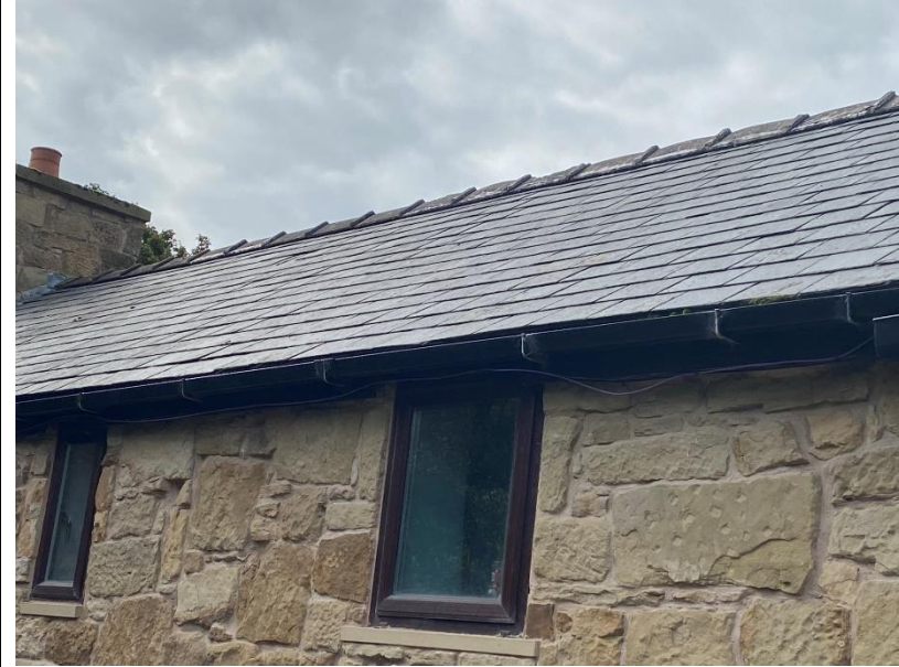
Eastern elevation of B1 (pictured above).
