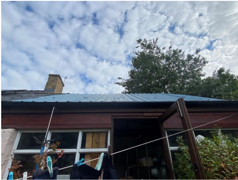
Western elevation of B1a (pictured above).
