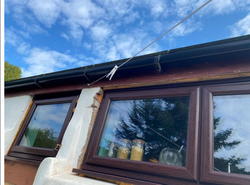
Western elevation of B1 (pictured above).
