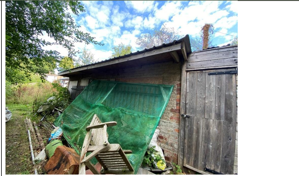
Western elevation of B3 (pictured above).
