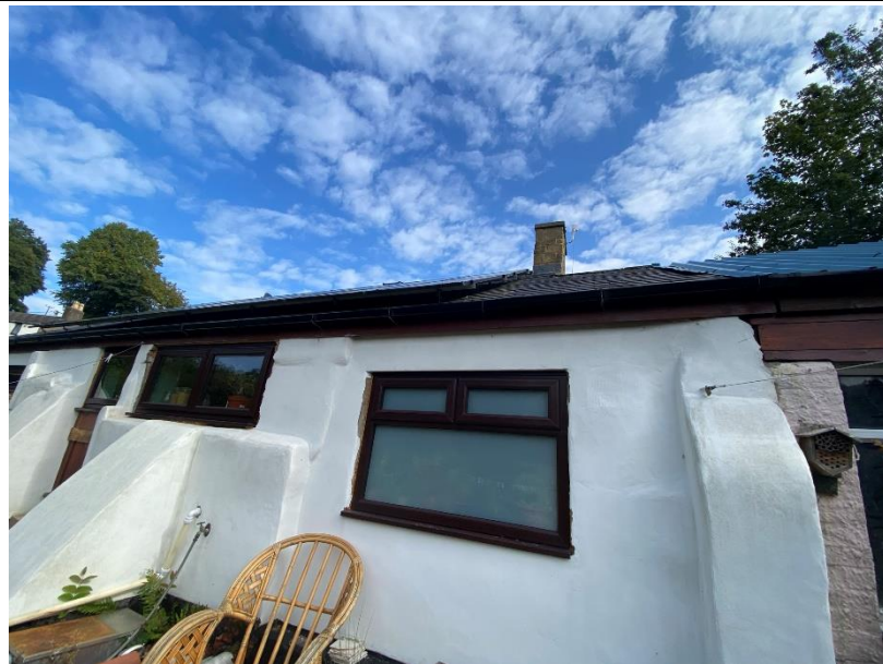
Western elevation of B1 (pictured above).
