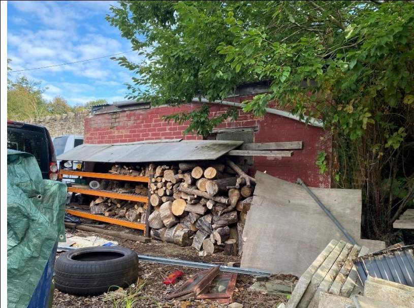
Western elevation of B2 (pictured above).
