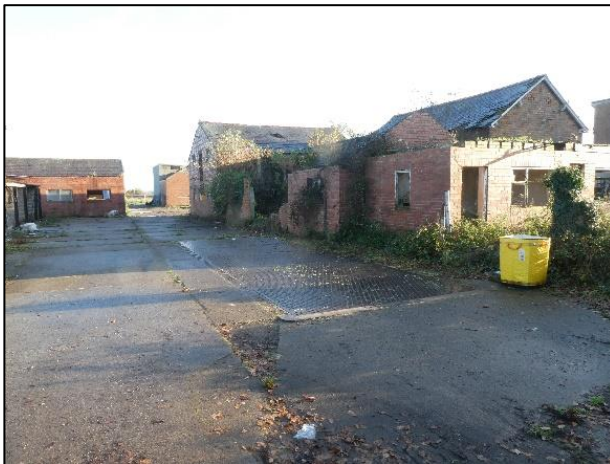
Weighbridge (to left of office building)
