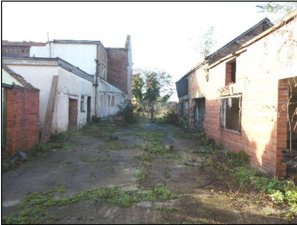
Former workshops and residential buildings
