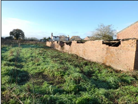
Partially cleared industrial buildings
