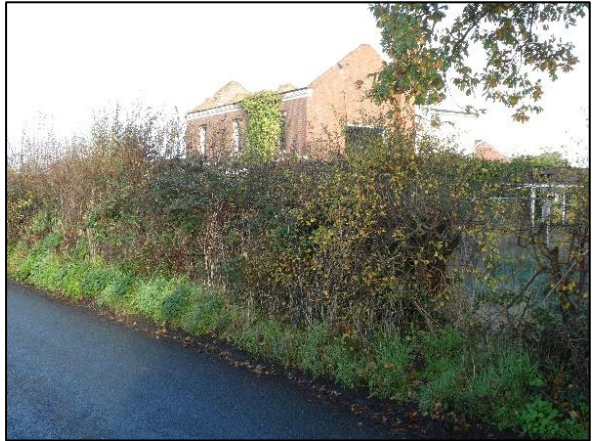
Former residential building to site frontage
