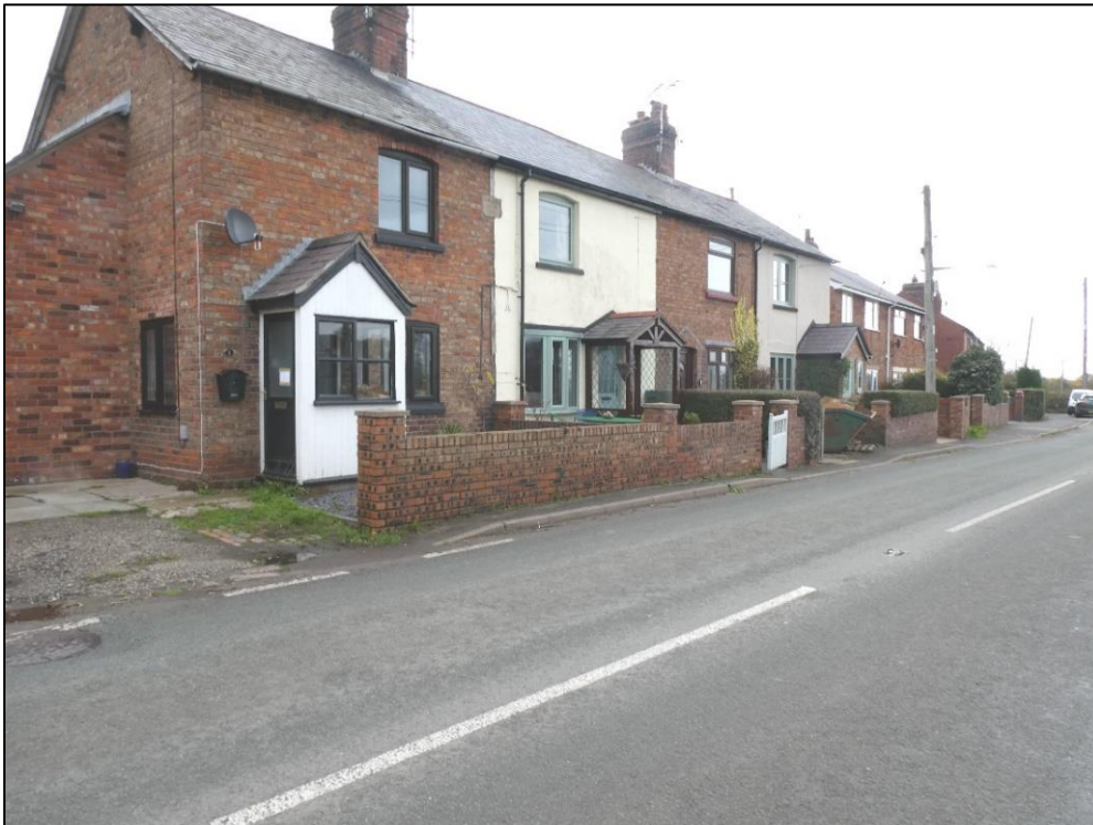
PHOTO 17 : GAMFORD ROAD AND ROSSETT ROAD COTTAGES 2
