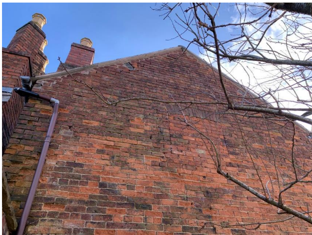
Plate 24 – Eastern elevation with potential roost features
