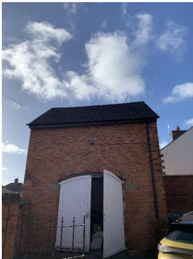
Plate 11 – North facing aspect of Building B2
