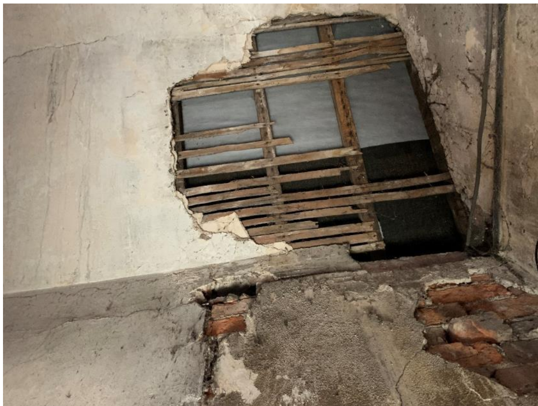
Plate 25 – Laff and plaster loft space with bitumen 1F present beneath
