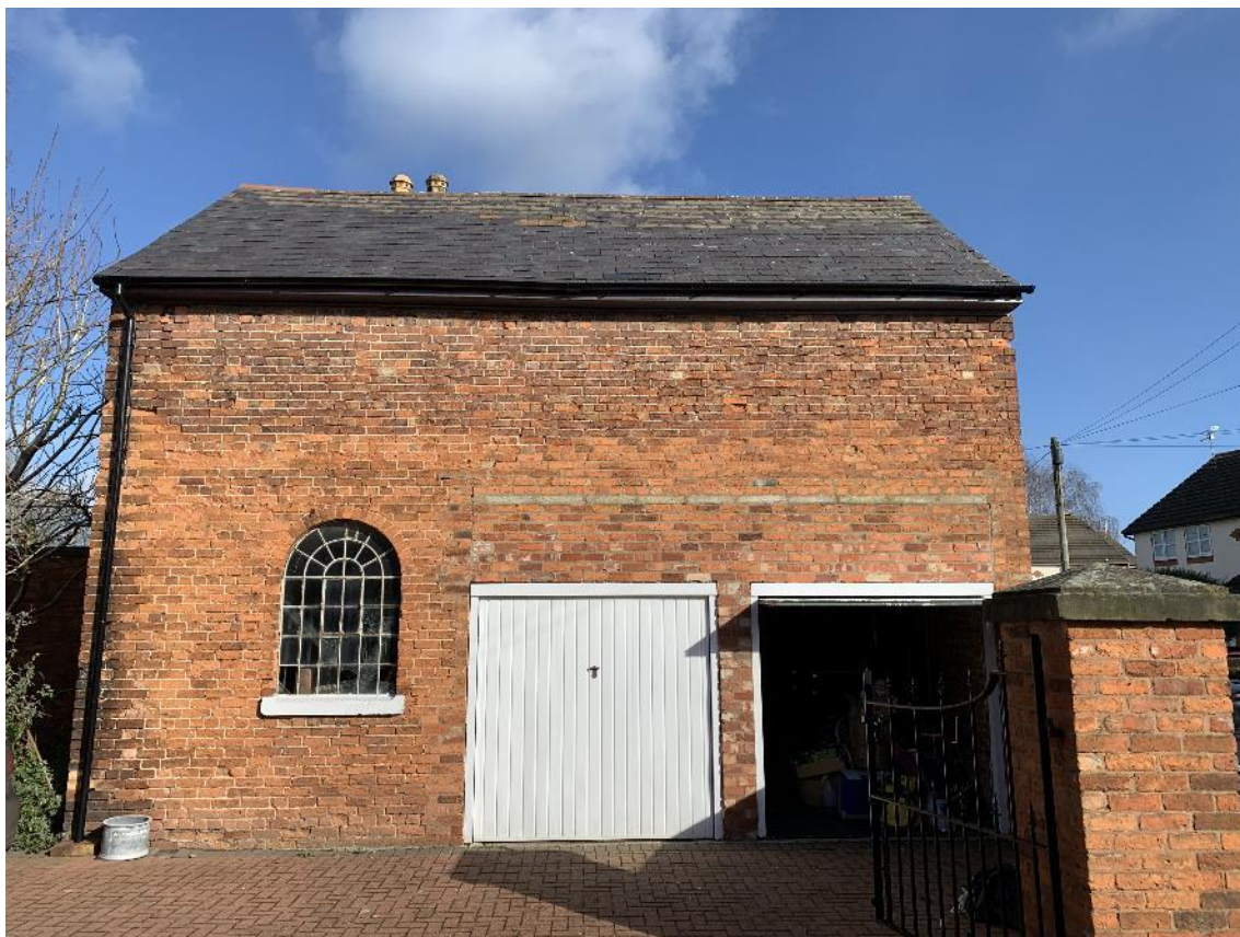
Plate 19 – Southern elevation of B3, showing steel doors
