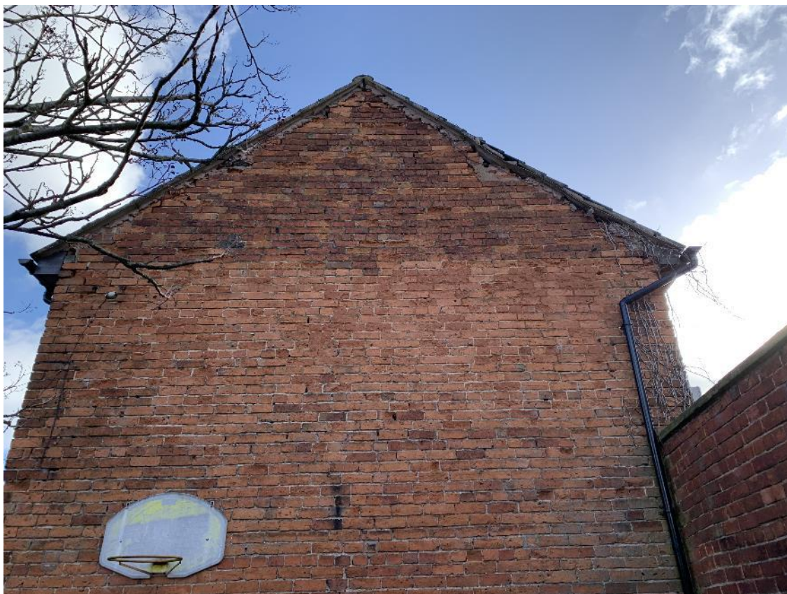
Plate 13 – West facing elevation, with a number of indicative entry points along gable
