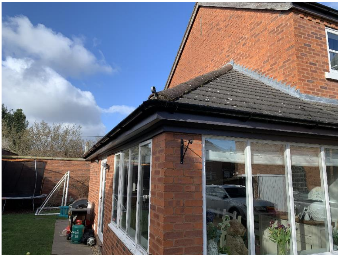
Plate 2 – Southern aspect showing single storey hipped rooved extension
