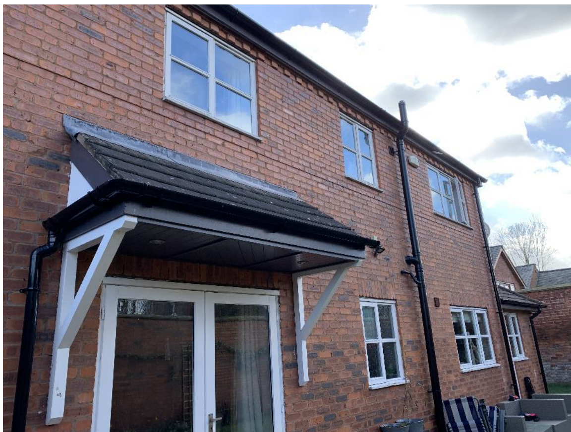
Plate 5 – West facing elevation
