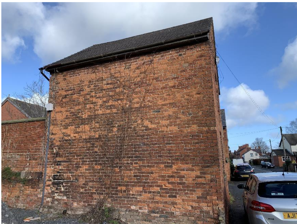
Plate 16 – Southern elevation of B2
