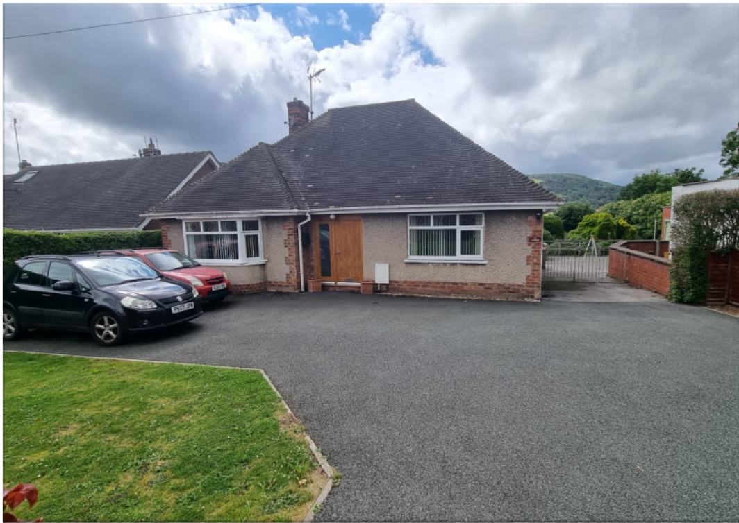
The Site looking from Park Road
