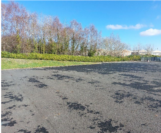
A view of the site and northern site boundary.
