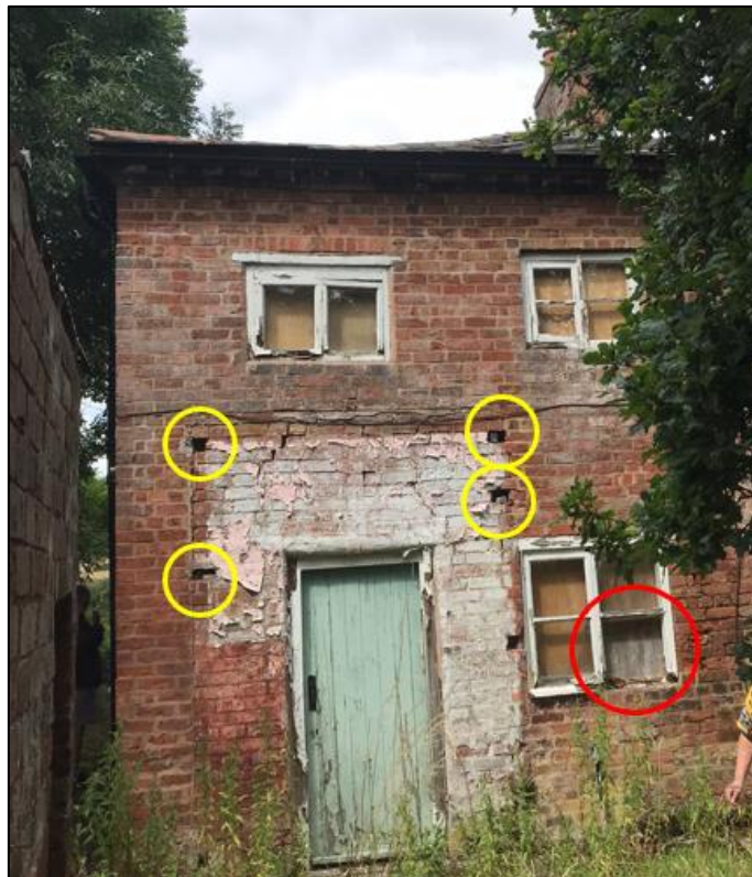
Plate 10. Gap above the front door
