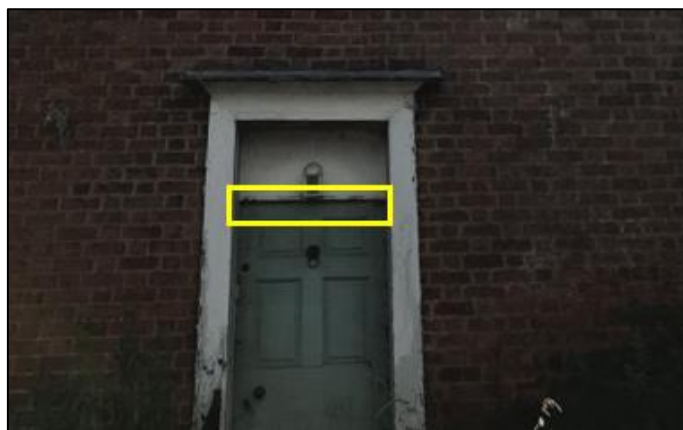
Plate 10. Gap above the front door
