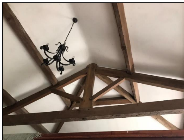
Plate 6. Exposed timber roof beams in lounge
