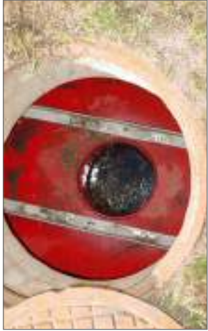
Fig. 7 View over center shaft into sediment storage zone.
