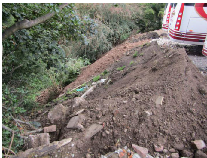
Photo 3: Soil and rubble on edge of infill.
