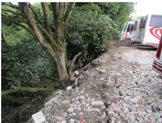
Photo 2: Sycamore with rubble piled around trunk.
