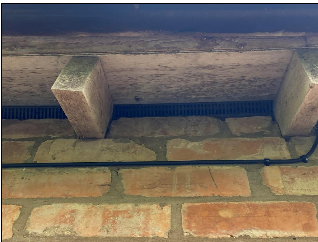
Plate 6 – Character of the eaves present throughout the majority of the dwelling; the presence of the pictured grate restricting access to the loft space by bats and/or birds
