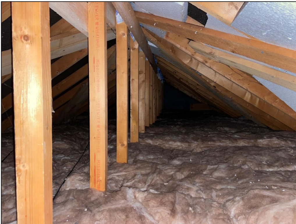
Plate 15 – Further character of the loft space above the dwelling
