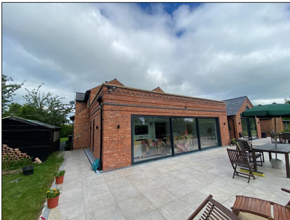
Plate 7 – Character of the rear of the dwelling / eastern elevation
