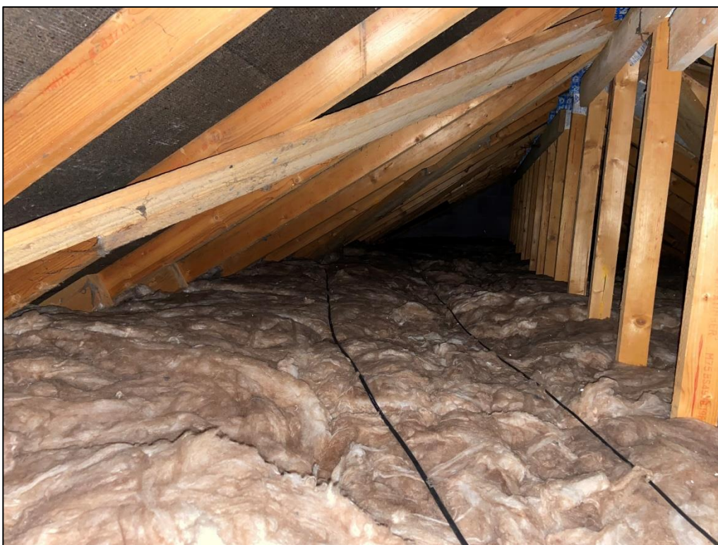
Plate 14 – Internal character of the loft space above the dwelling
