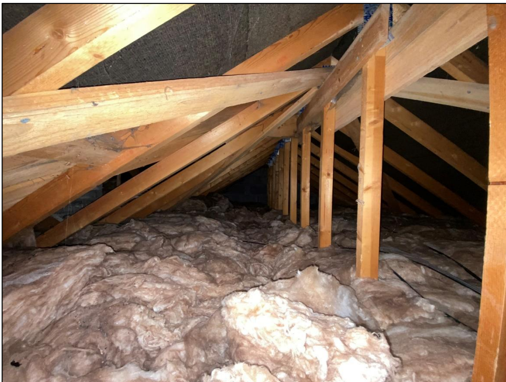
Plate 16 – Further character of the loft space above the dwelling
