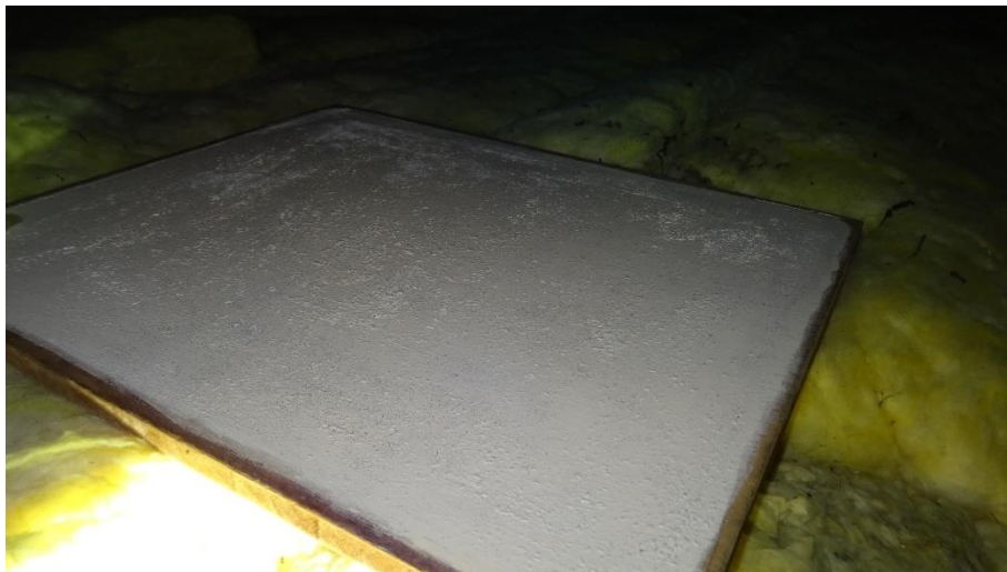
Figure 4.5. Loft surfaces free of bat droppings
