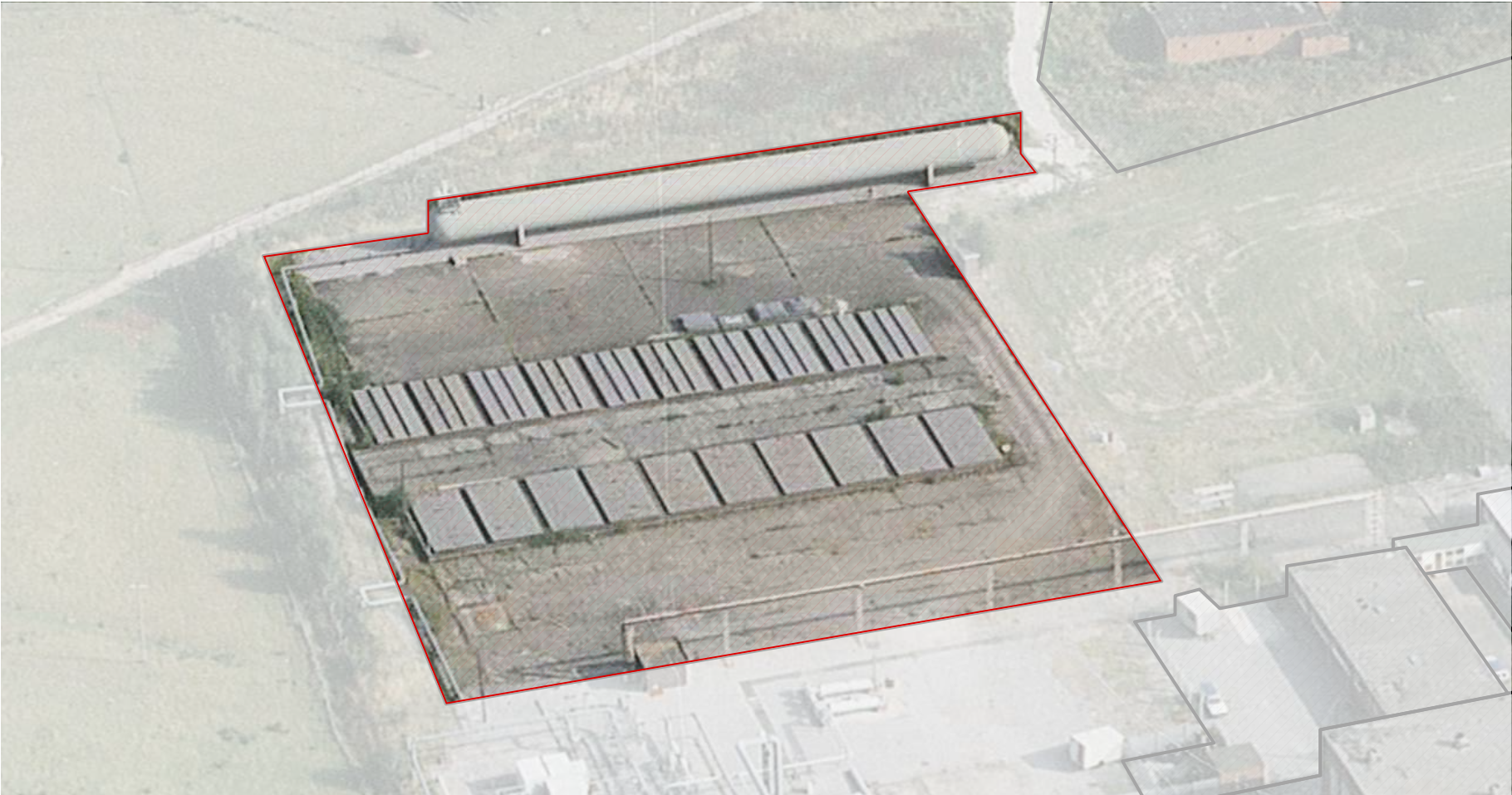
Purifiers - highlighted aerial image
