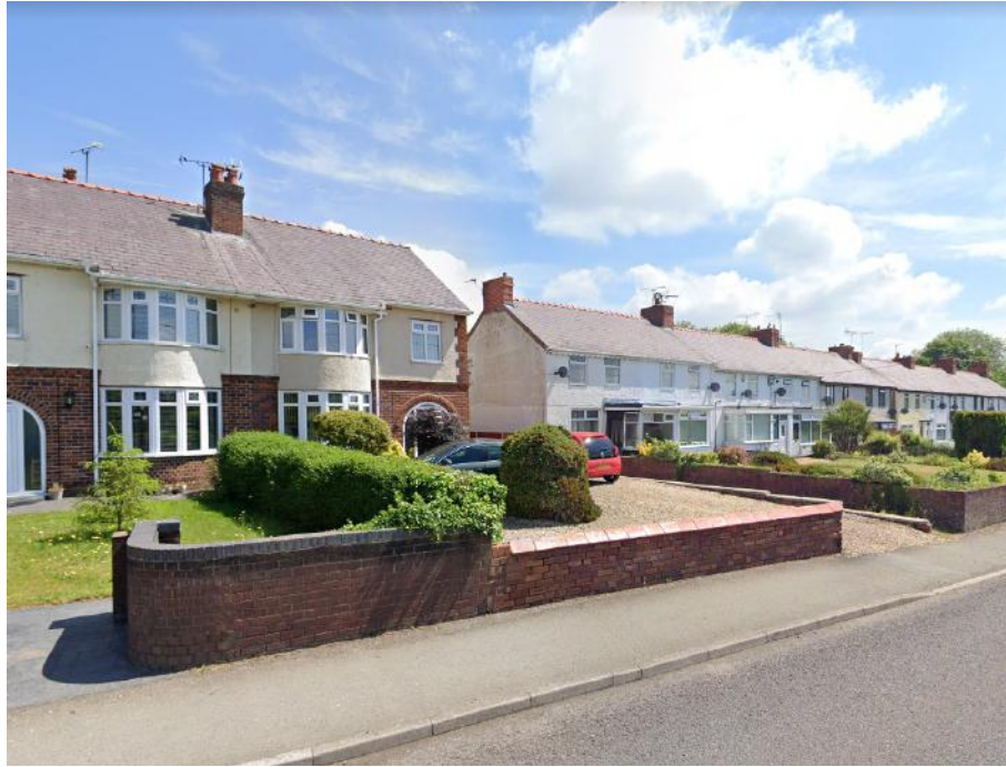
Houses that overlook the site on Berse Rd
