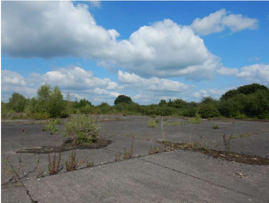
Photograph 3 – The existing hardstanding in the south-eastern corner of the site.
