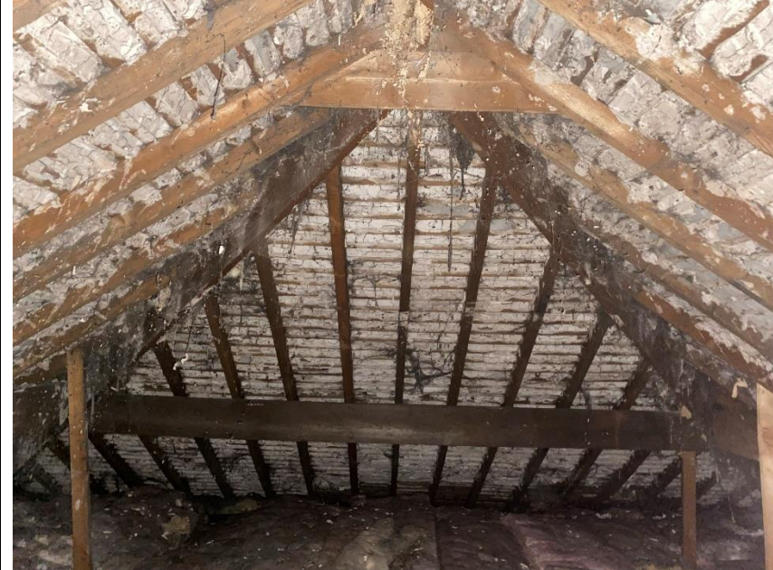
Internal loft space of B1 (pictured above).
