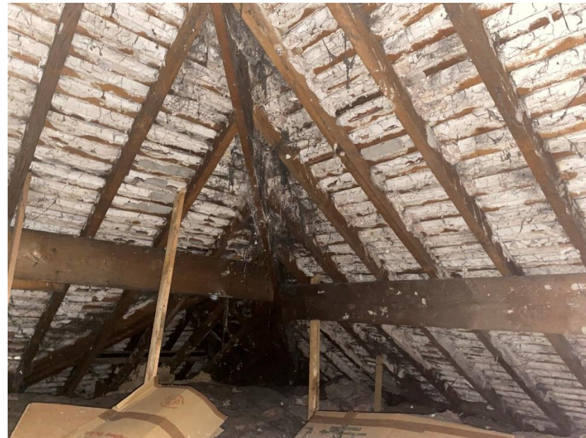
Internal loft space of B1 (pictured above).
