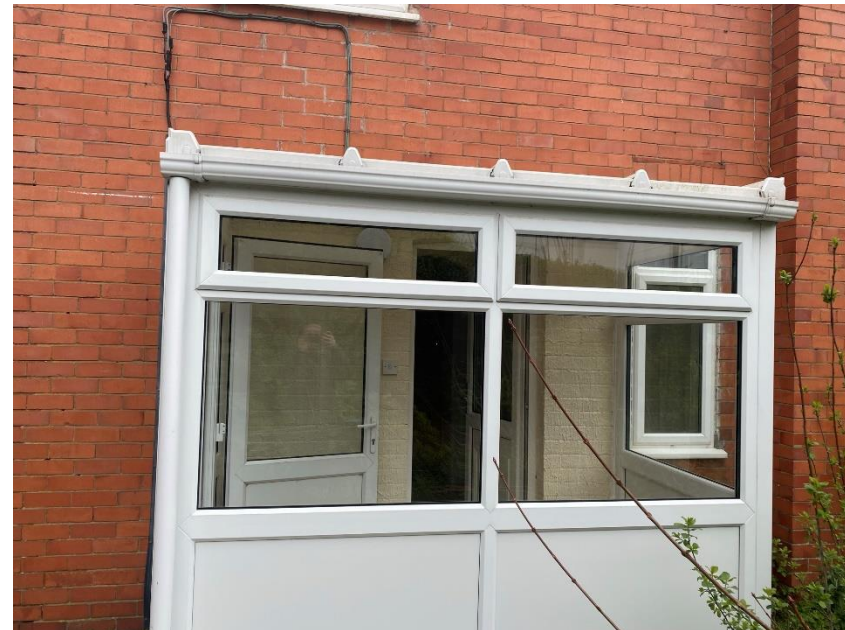
Single-storey extension on western elevation of B1 (pictured above).
