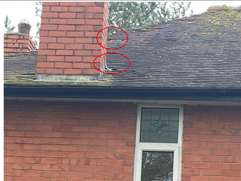
Close-up of the roof structure on northern elevation of B1 (pictured above).
