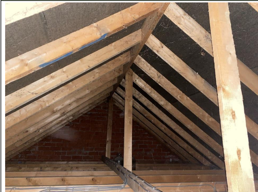
Internal loft space of B2 (pictured above).
