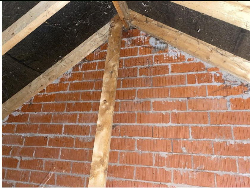
Internal loft space of B2 (pictured above).
