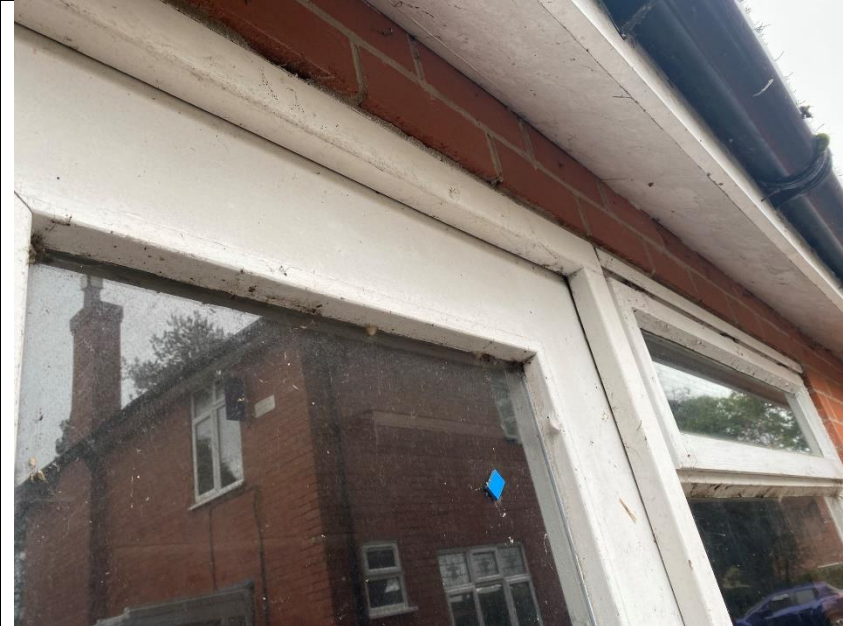
Close-up of eaves along southern elevation of B2 (pictured above).
