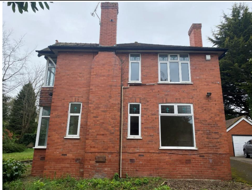
Eastern elevation of B1 (pictured above).
