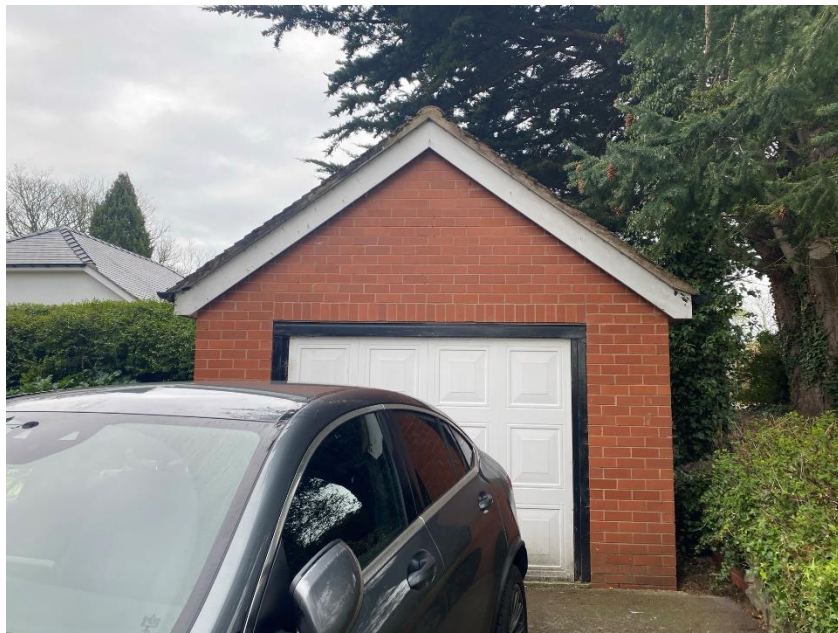
Eastern elevation of B2 (pictured above).
