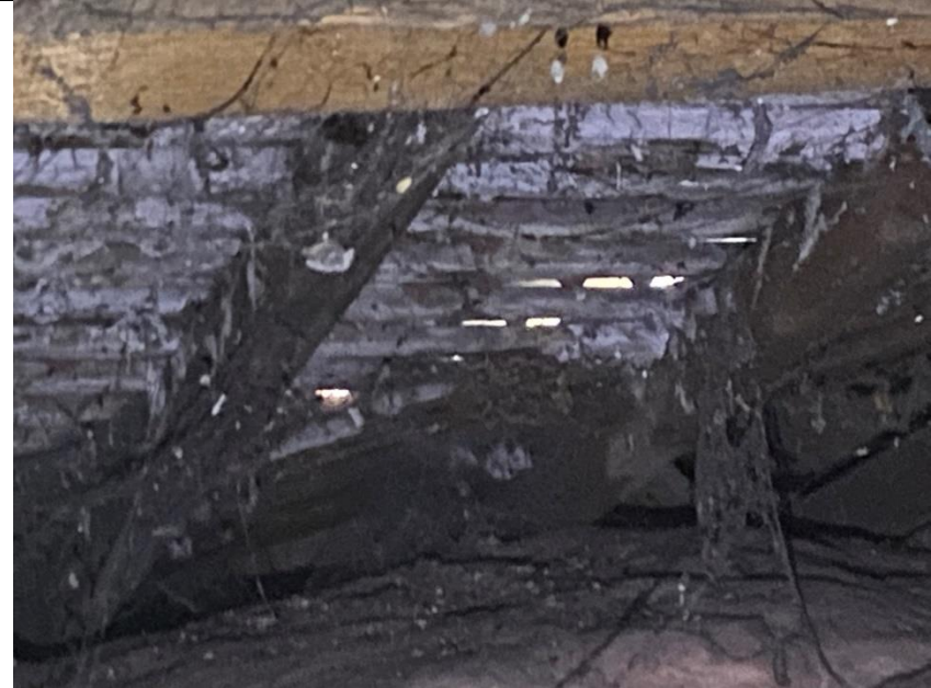
Internal loft space of B1 (pictured above).
