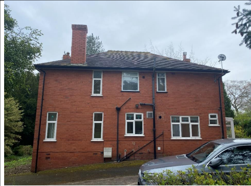
Northern elevation of B1 (pictured above).
