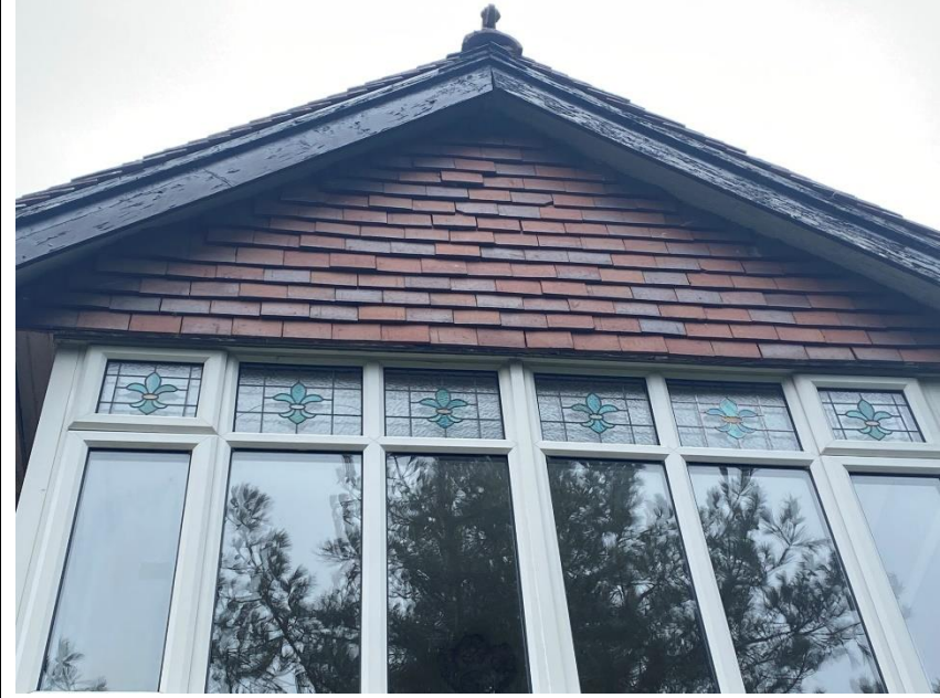
Close-up of hanging tiles on southern elevation of B1 (pictured above).
