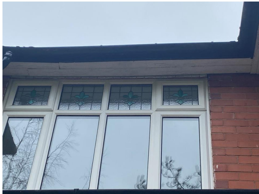
Close-up of eaves on southern elevation of B1 (pictured above).
