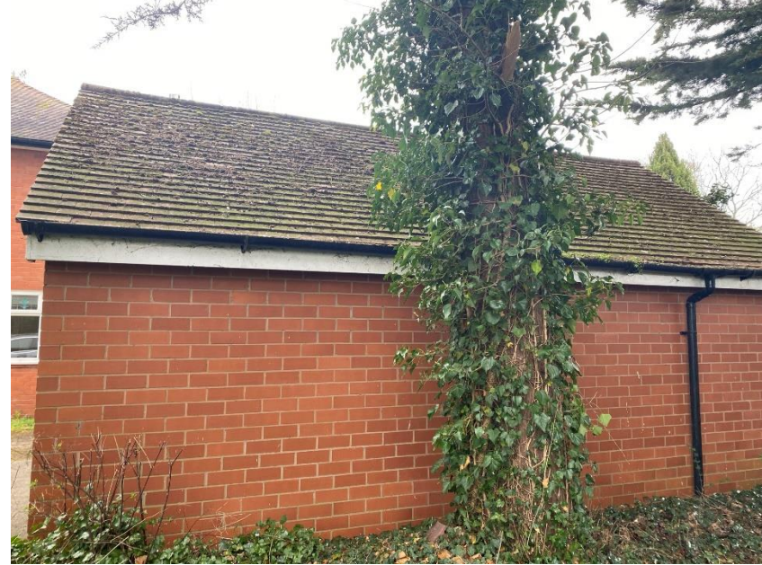
Northern elevation of B2 (pictured above).
