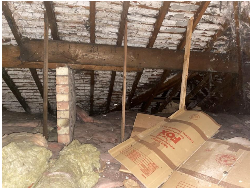
Internal loft space of B1 (pictured above).
