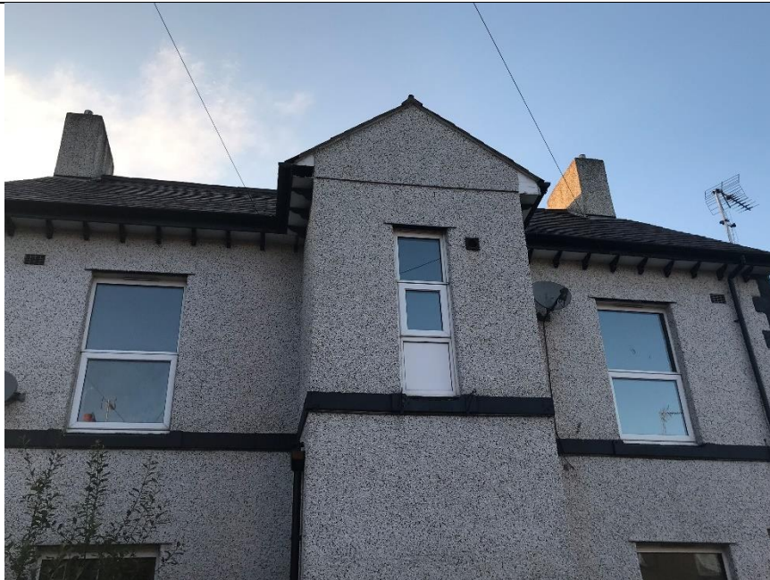
Photograph 2: Rear of the site, taken from the garden of the property.
