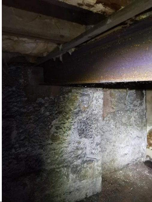
Photograph 17: The steel beam in the basement.
