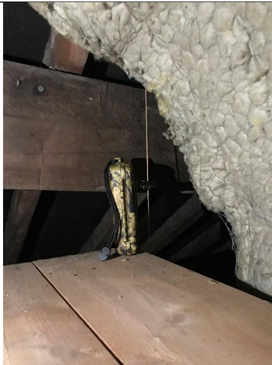
Photograph 22: The static detector in situ in the loft space.
