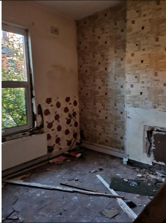
Photograph 15: An example of the interior rooms in the property.
