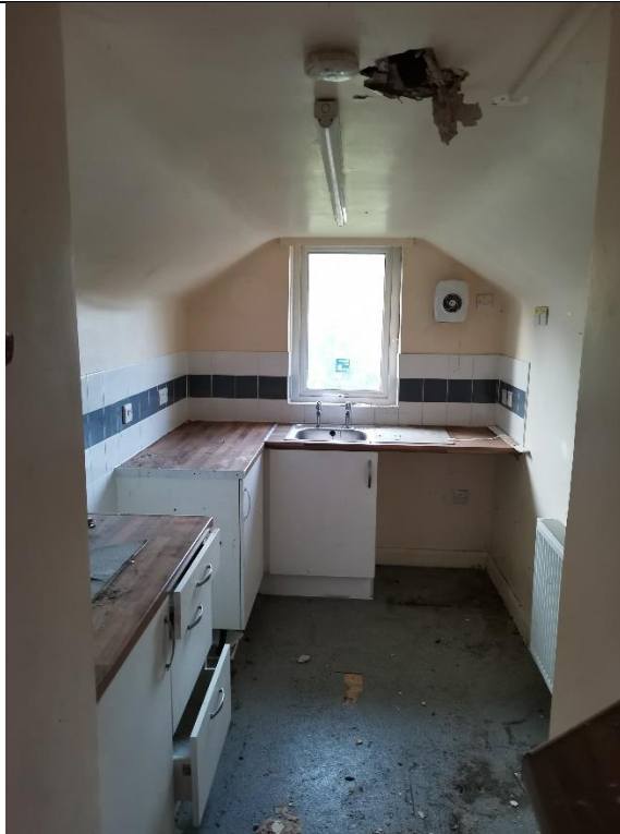
Photograph 14: An example of the interior rooms in the property.
