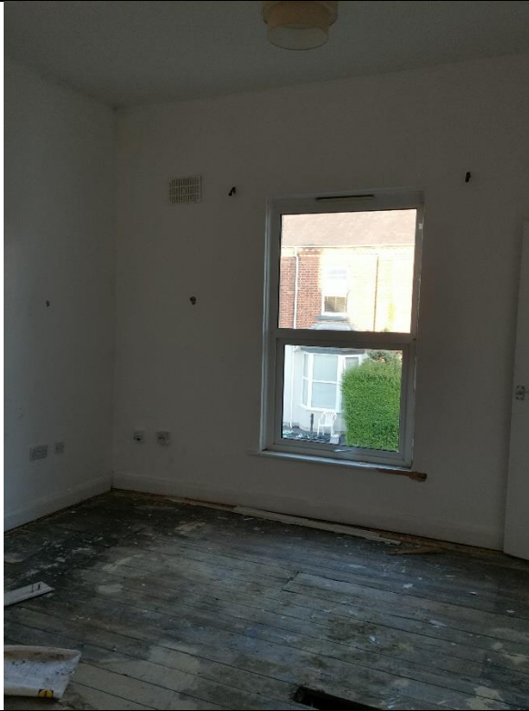
Photograph 11: An example of the interior rooms in the property.
