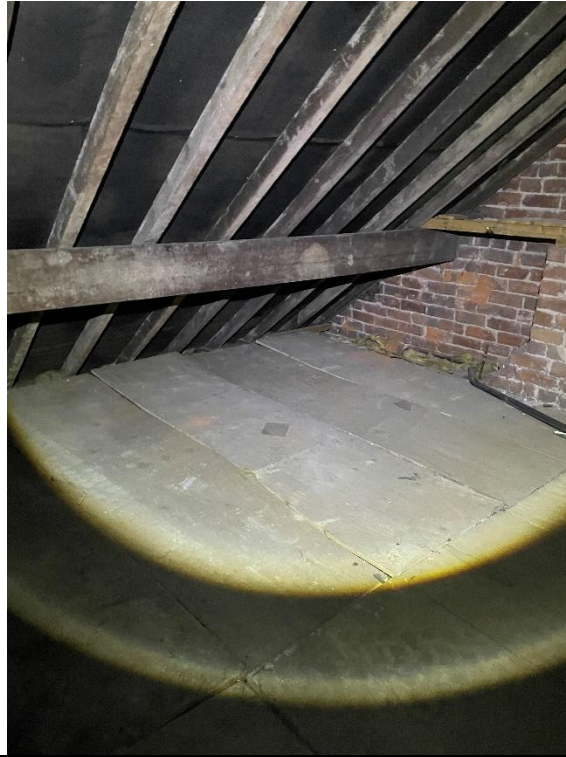
Photograph 21: The loft space, showing the rafters, purlin, bitumen backed tiles, brick east gable wall and floor boards.
