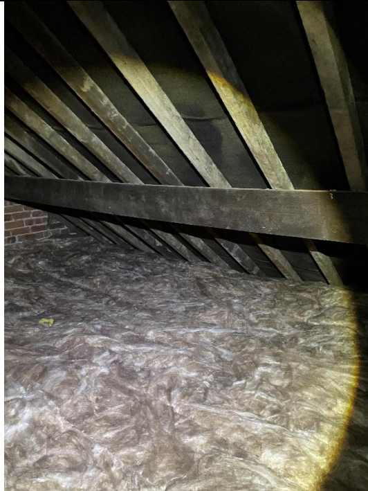
Photograph 20: The loft space, showing the rafters, purlin, bitumen backed tiles, brick eastern gable wall and loft insulation.
