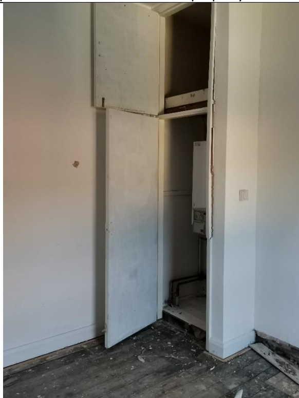
Photograph 12: An example of the interior rooms in the property.
