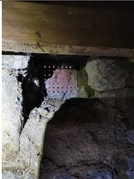
Photograph 18: The air vent/brick in the basement.
