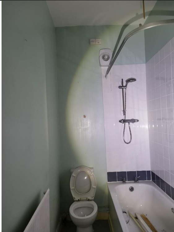
Photograph 13: An example of the interior rooms in the property.
