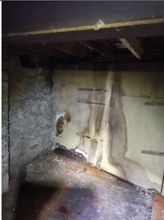
Photograph 16: Basement showing the stone floor and walls.
