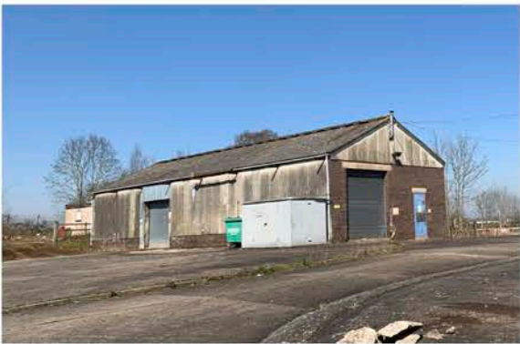
Welding workshop & Store A1 - Exterior Image
