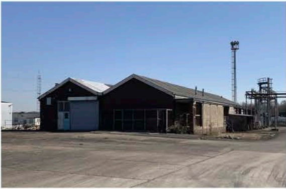
Welding workshop & Store A2 - Exterior Image
