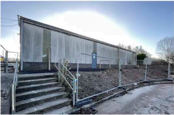
Welding workshop & Store A1 - Exterior Image
