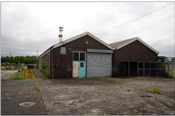
Welding workshop & Store A2 - Exterior Image
