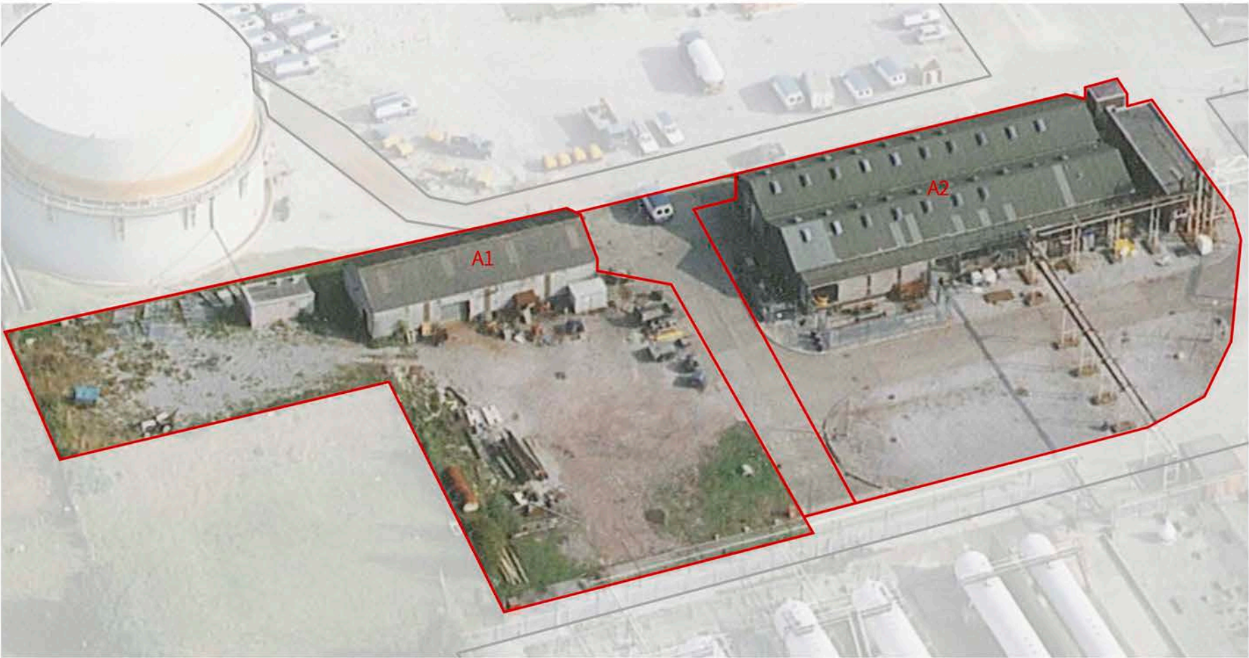
Welding workshop & Store - highlighted aerial image
