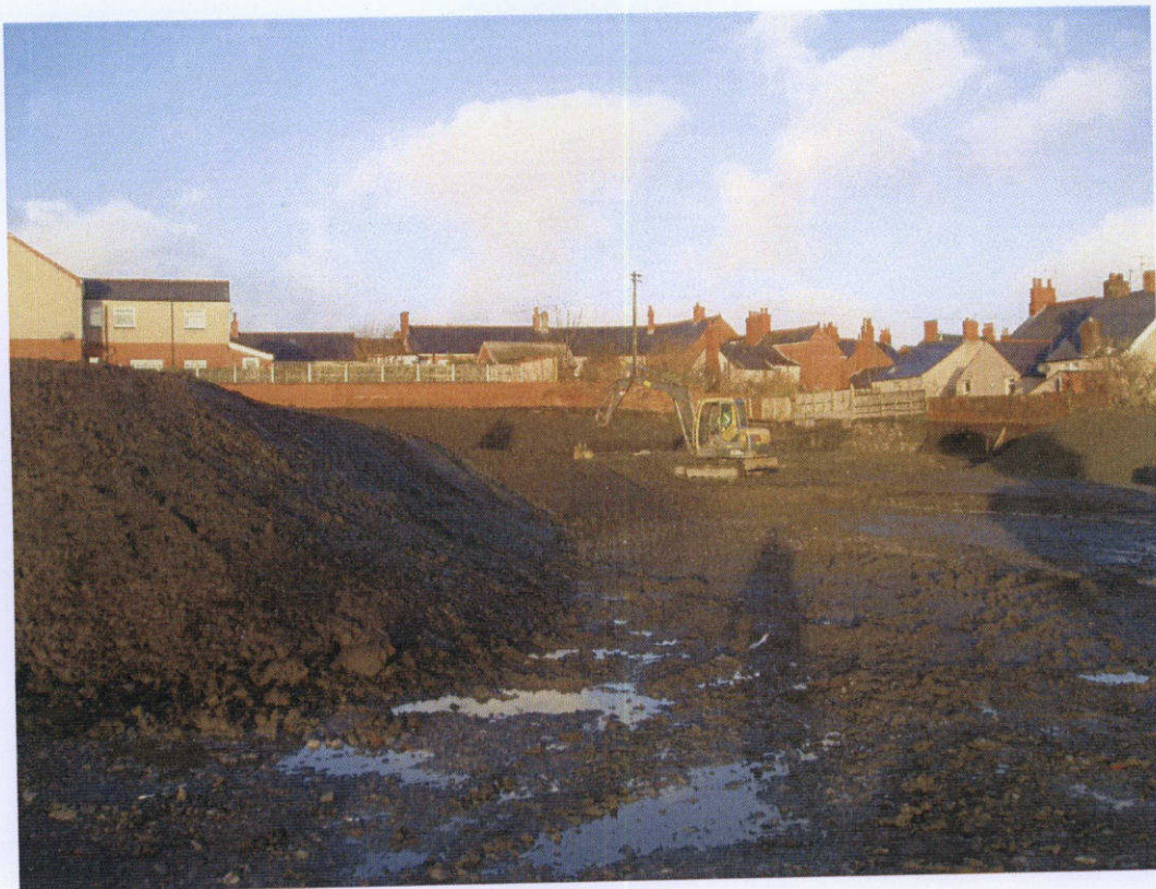
Photograph 8 Showing main section of site looking west
