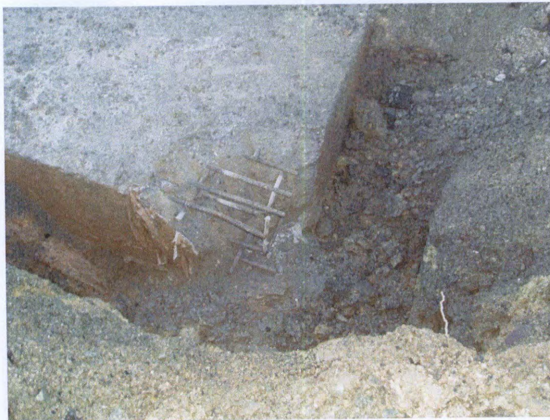
Photograph 5 Showing reinforcement in cap
