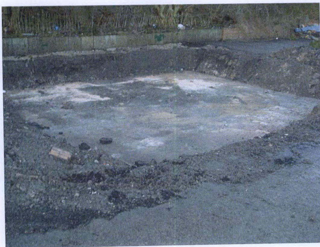
Photograph 6 Showing shaft cap
