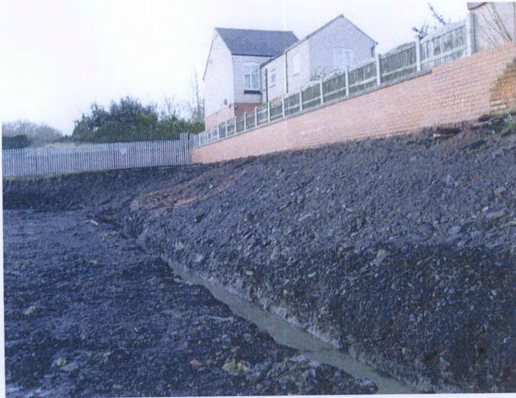
Photograph 1 Showing reduced ground levels along western site boundary, looking south
