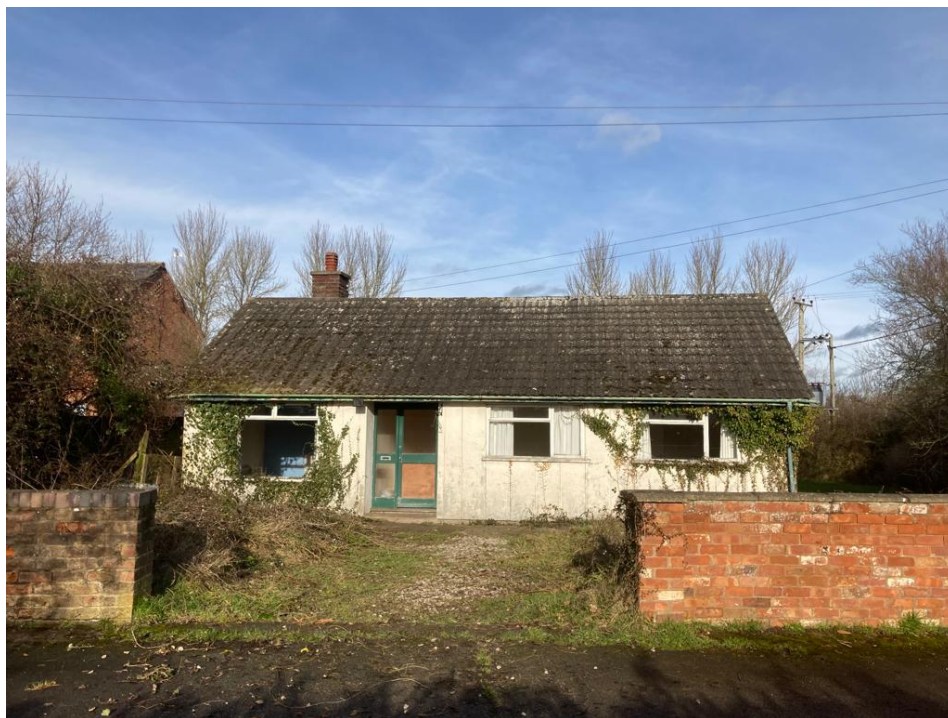
Image 1 - existing property of The Bungalow, Cae Lica Farm
