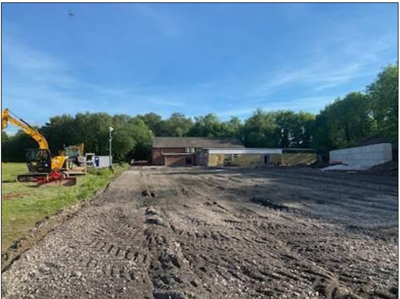
Plate 5-1: Photograph of the site area with hardstanding removed.
