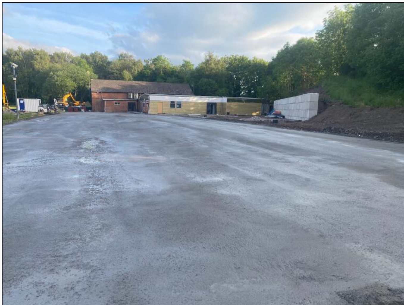
Plate 5.3 – Photograph of the site area after concrete soil mixing.
