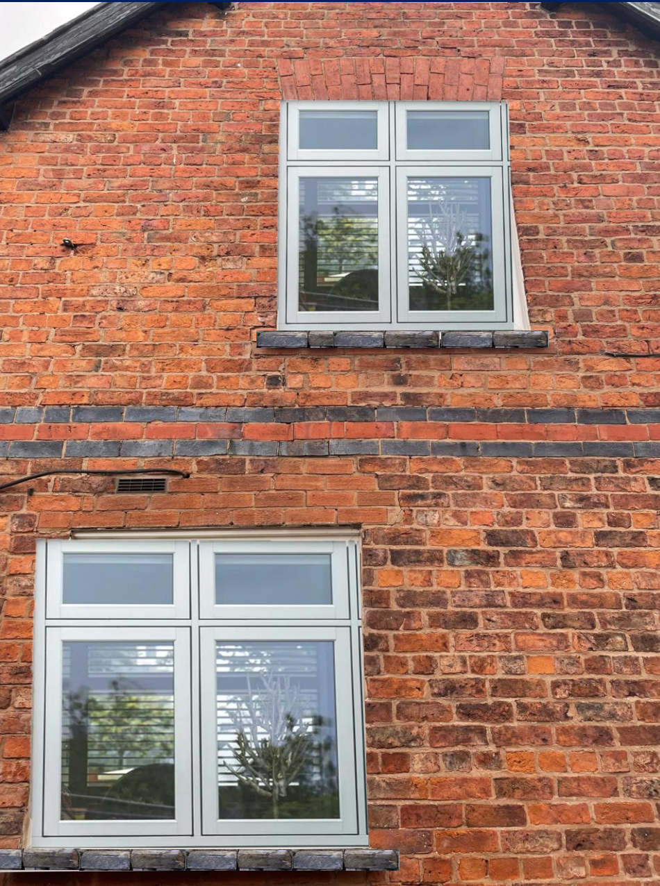
Plus additional replacement of blue plinth stretcher bricks to match historic band of bricks on wall
