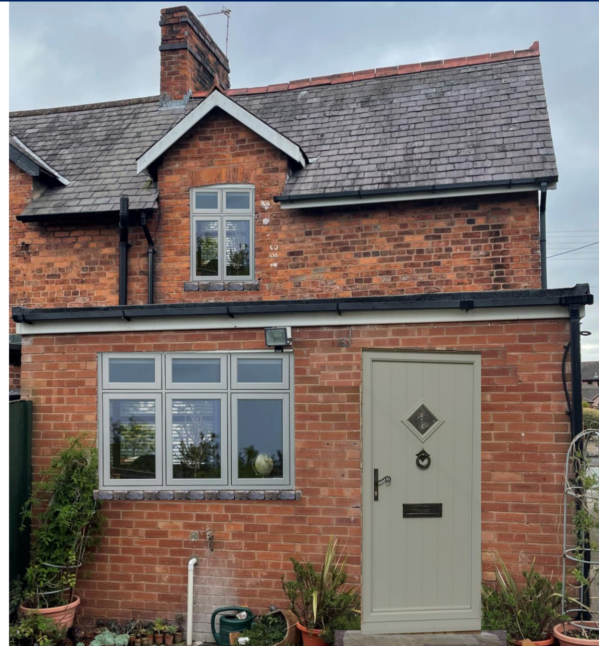
Plus additional replacement of blue plinth stretcher bricks to match historic band of bricks on wall
