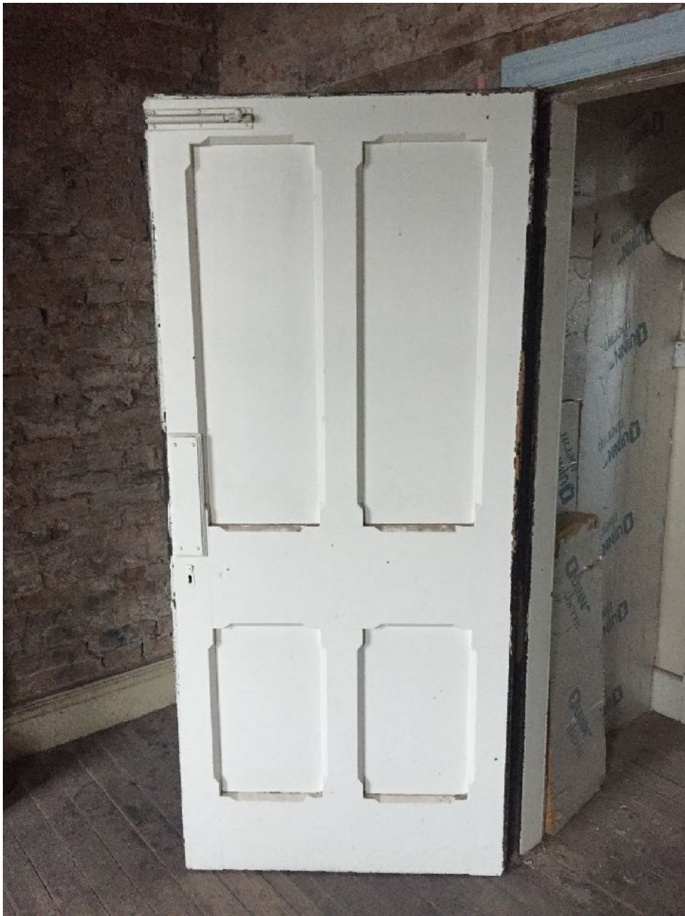
Victorian 4-panelled door.
