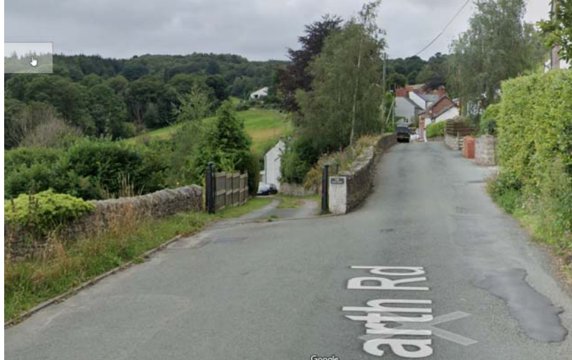
Image 12: Existing access to The Cottage off Garth Road, to be altered.
