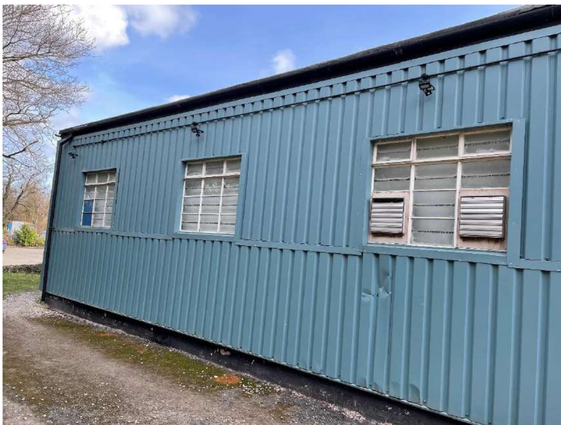
Photograph 3. The north-western aspect of Building 3.
