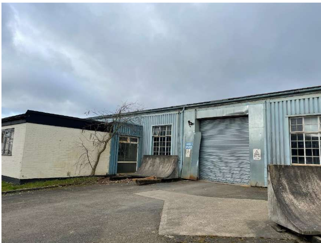
Photograph 11. The south-eastern aspect of Building 4.
