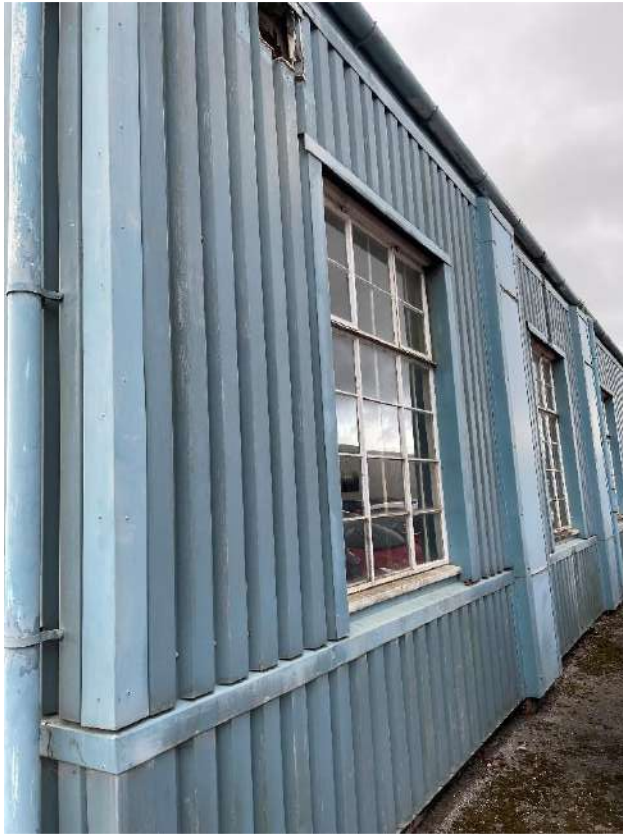
Photograph 9. The north-western aspect of Building 4.
