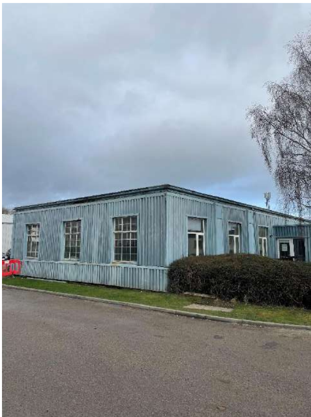
Photograph 8. The south-western aspect of Building 4.
