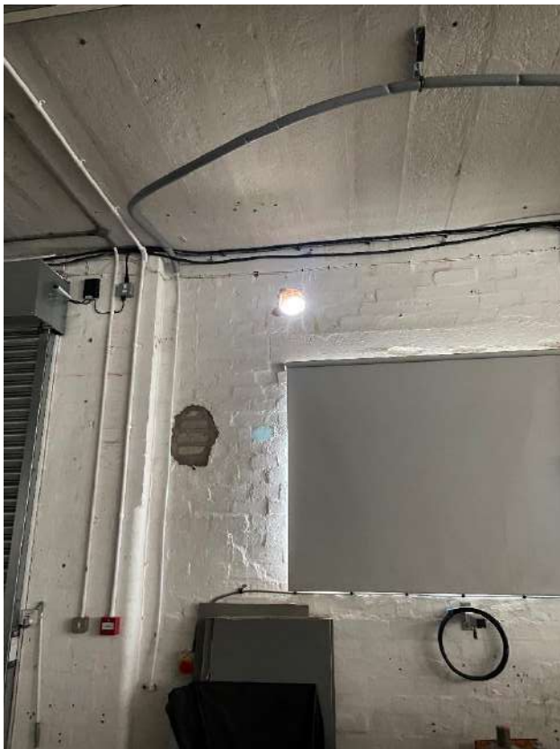
Photograph 22. An access point into Building 3.
