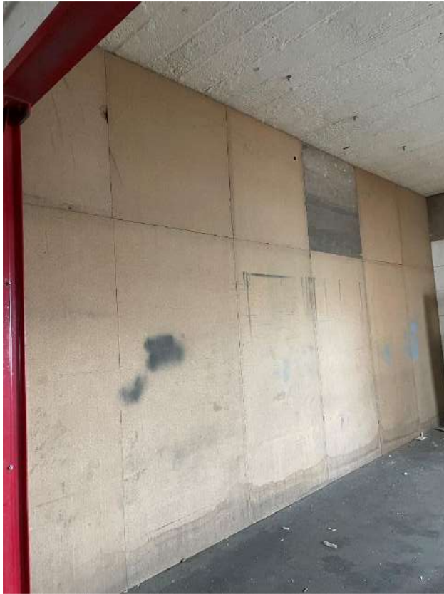
Photograph 25. The interior of Building 4.
