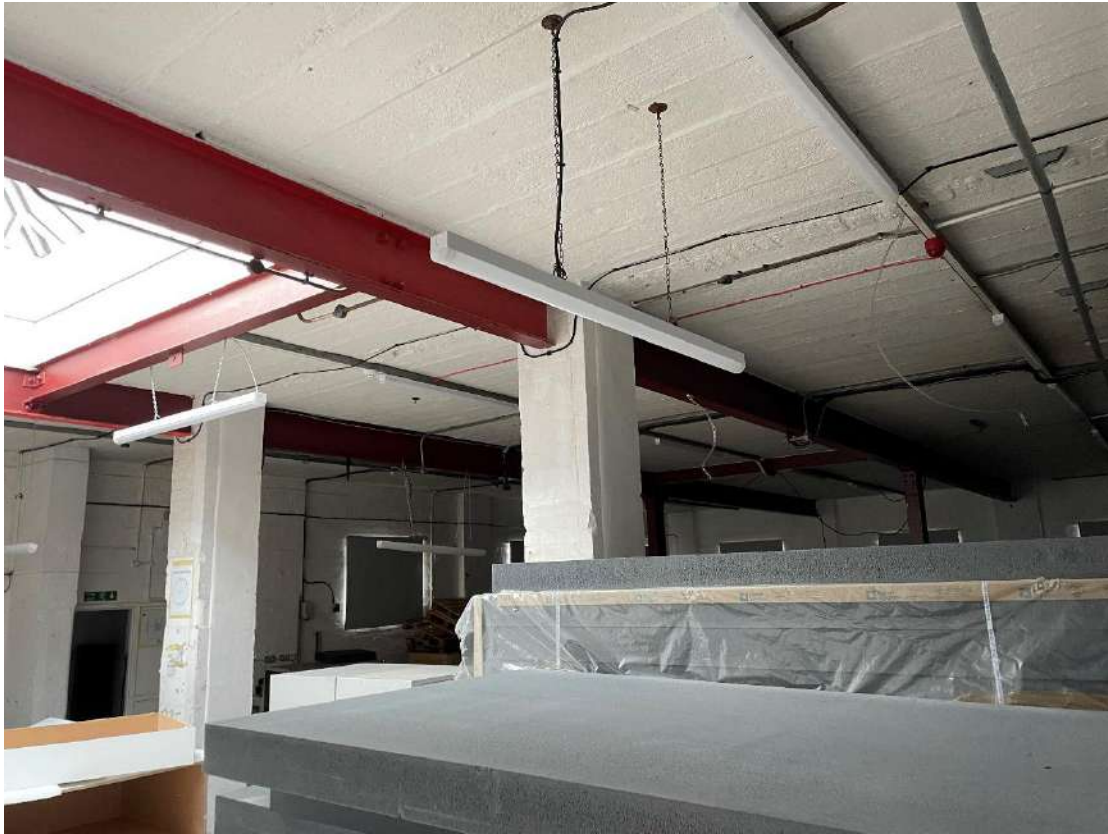
Photograph 21. The brick columns inside Building 3.
