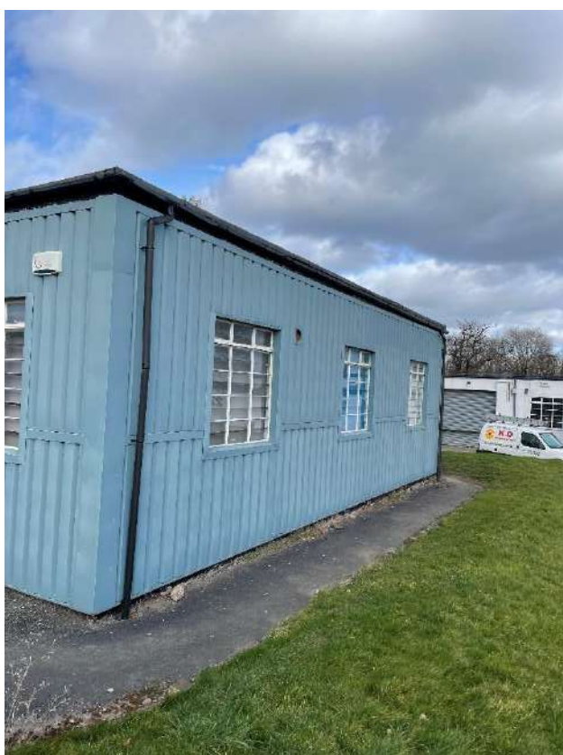
Photograph 2. The south-eastern aspect of Building 3.
