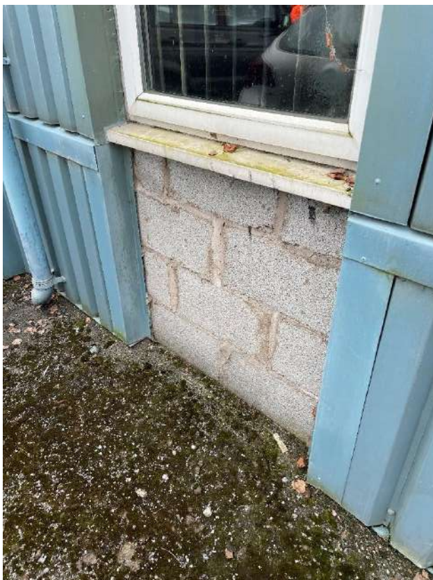
Photograph 14. A breezeblock wall on the north-western aspect of Building 4.
