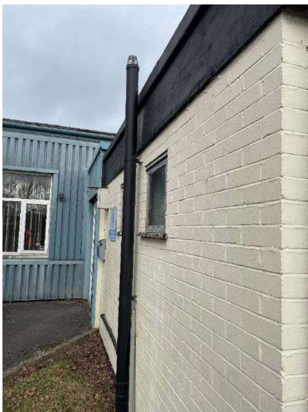
Photograph 18. The single-storey brick extension on the south-eastern aspect of Building 4.
