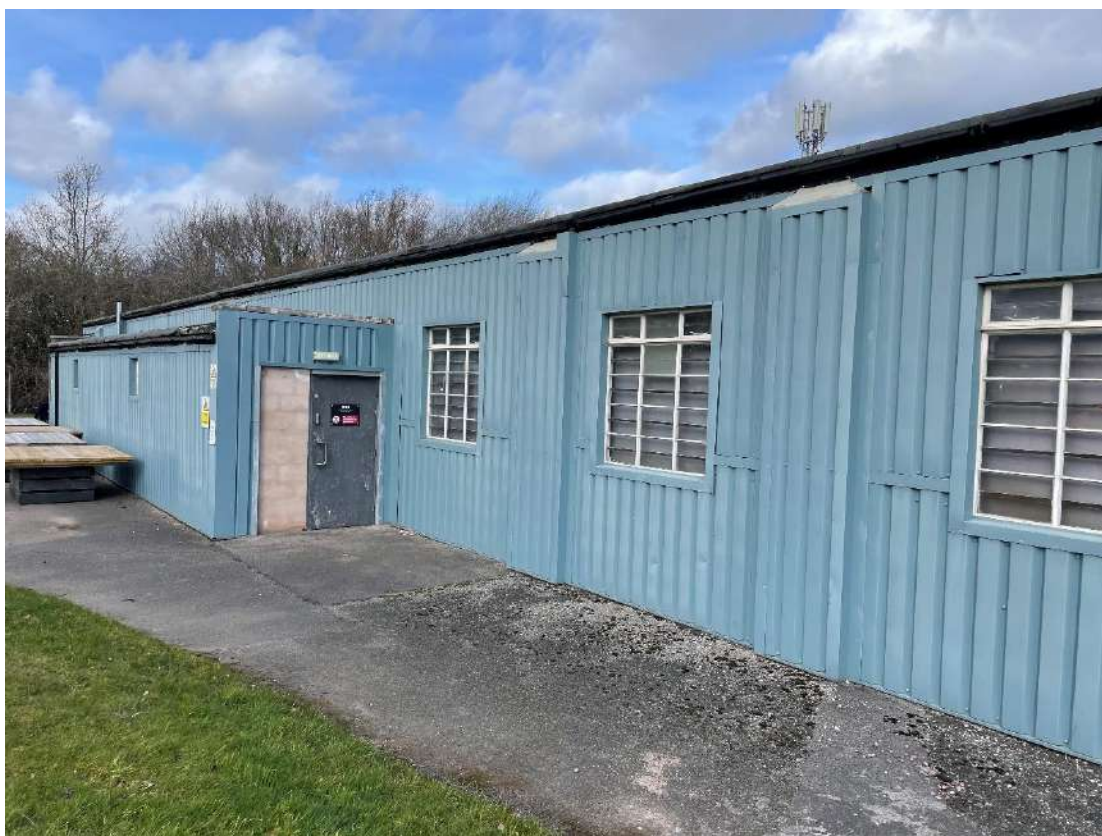
Photograph 1. The south-western aspect of Building 3.
