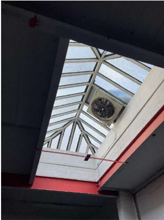
Photograph 23. A skylight on Building 3.
