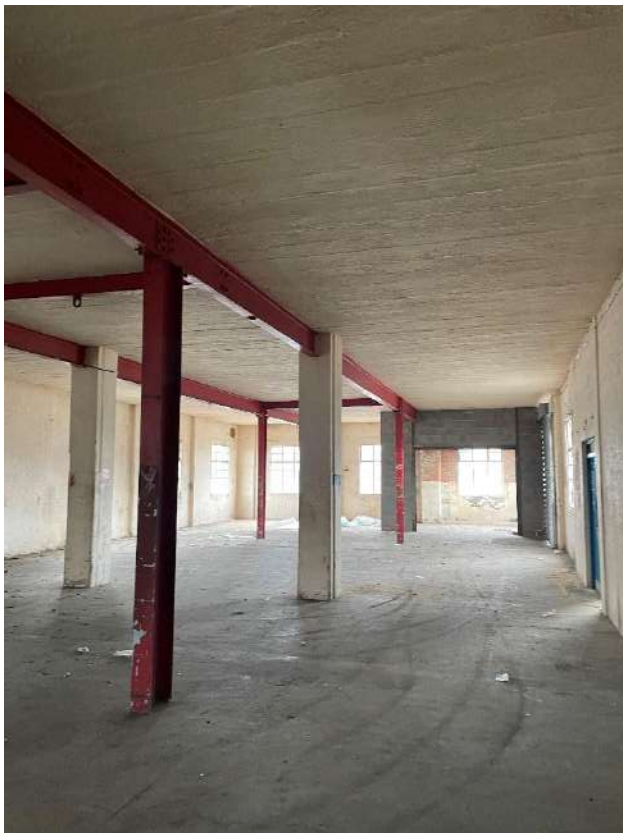
Photograph 24. The interior of Building 4.
