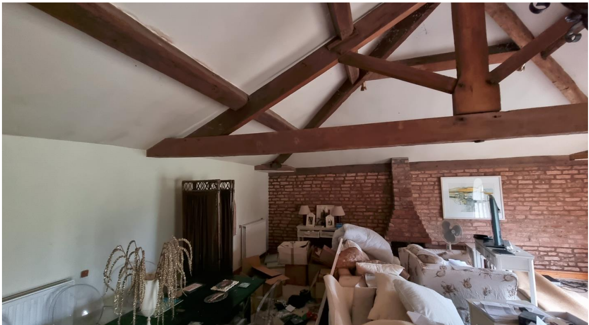
Pl.3: Part of the first-floor inserted into the chapel section, showing part of the roof structure.
