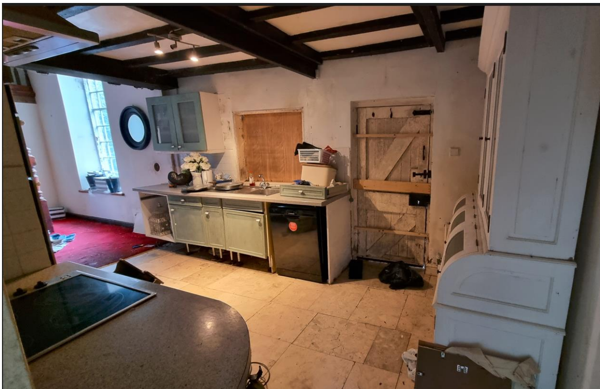
Pl.5: View from within the remodelled ground-floor of the former minister's house through the site of the cross-wall between it and the former chapel section beyond.
