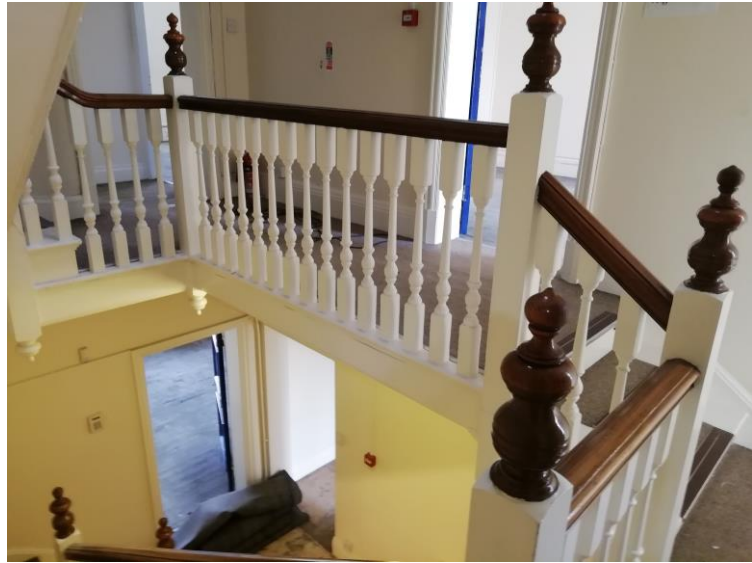
Fig.9 – Original bank entrance Fig.10 – Staircase balustrade to be retained
