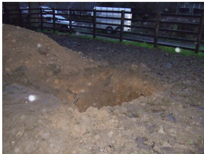
Percolation test pit, January 2021
