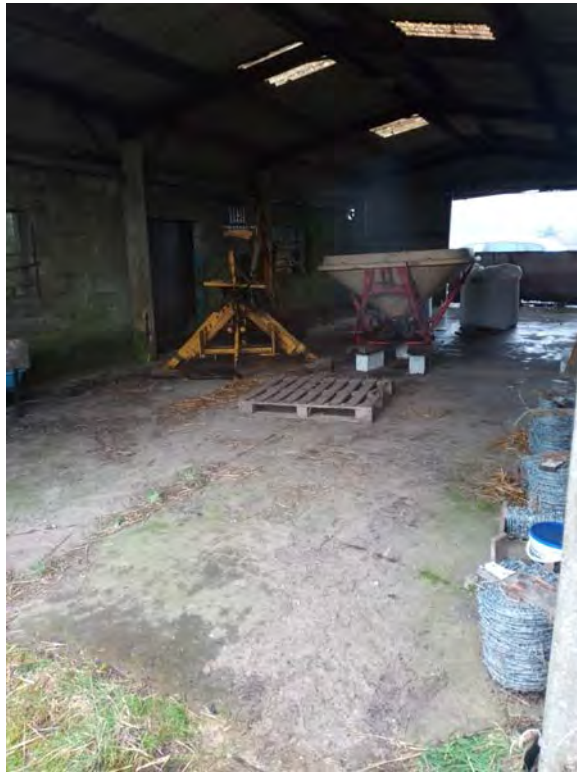
Photo 3: Building in the north west of the Site.
