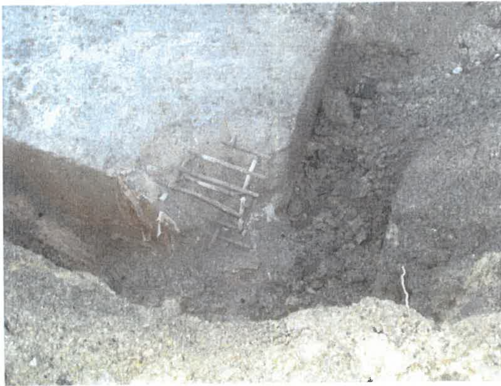
Photograph 5 Showing reinforcement in cap
