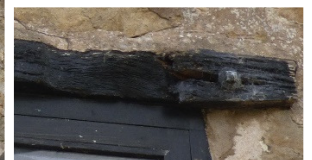
Lintel over W.1.4
