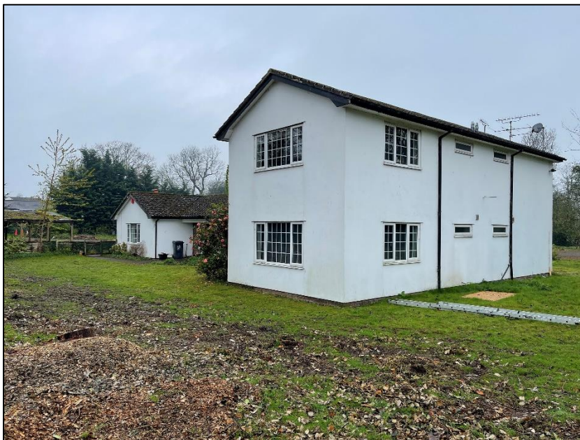
Photograph 10 showing the front of the dwelling
