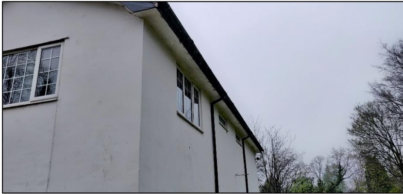
Photograph 13 showing the soffits at the two-storey section
