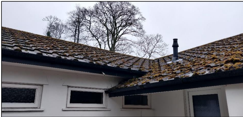
Photograph 11 showing the roof at the rear as well as lead flashing
