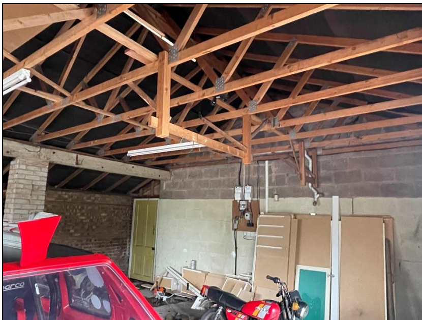
Photograph 16 showing the interior roof of the garaging
