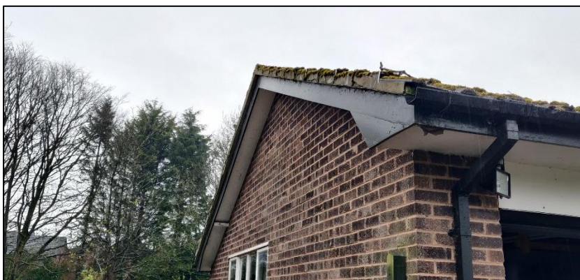
Photograph 12 showing the roof edge at the garage
