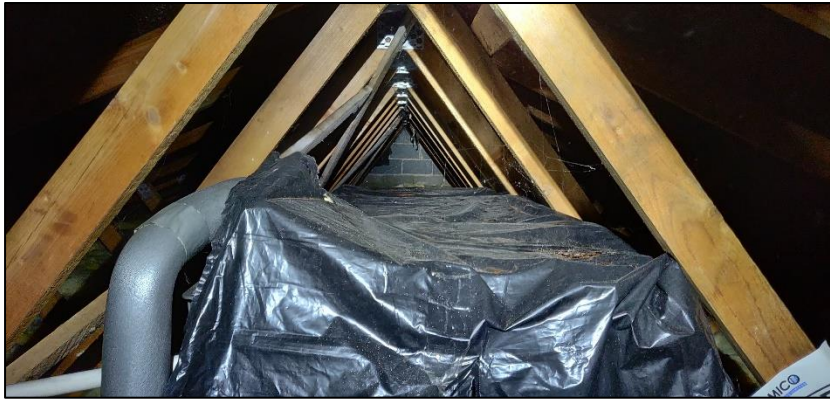
Photograph 15 showing the roof void above the double-storey part of the dwelling
