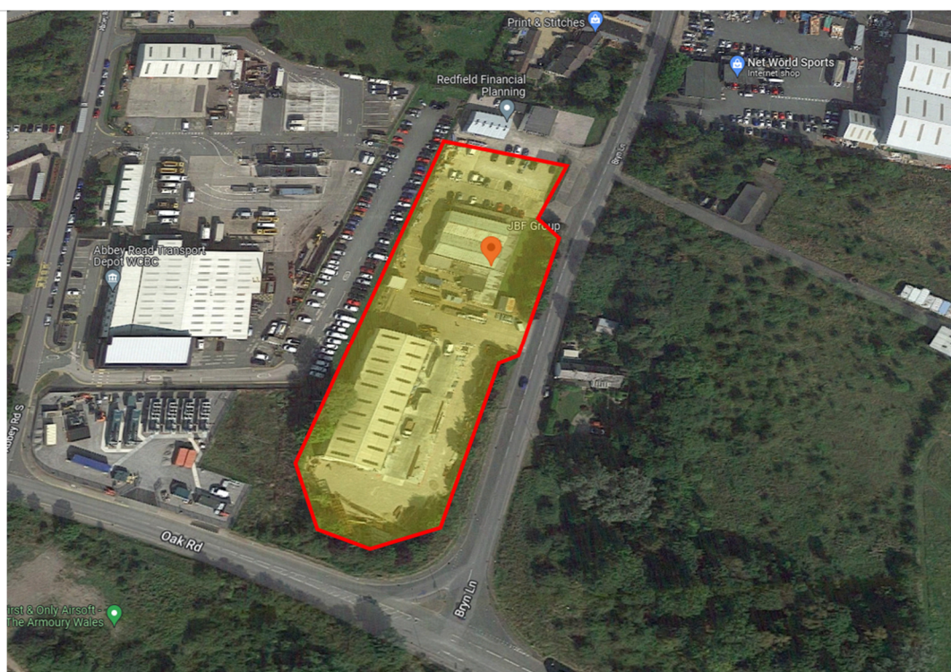
Aerial View of the JBF Group site.
