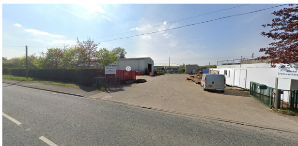
View of Gate 1 from Bryn Lane – Deliveries Only
