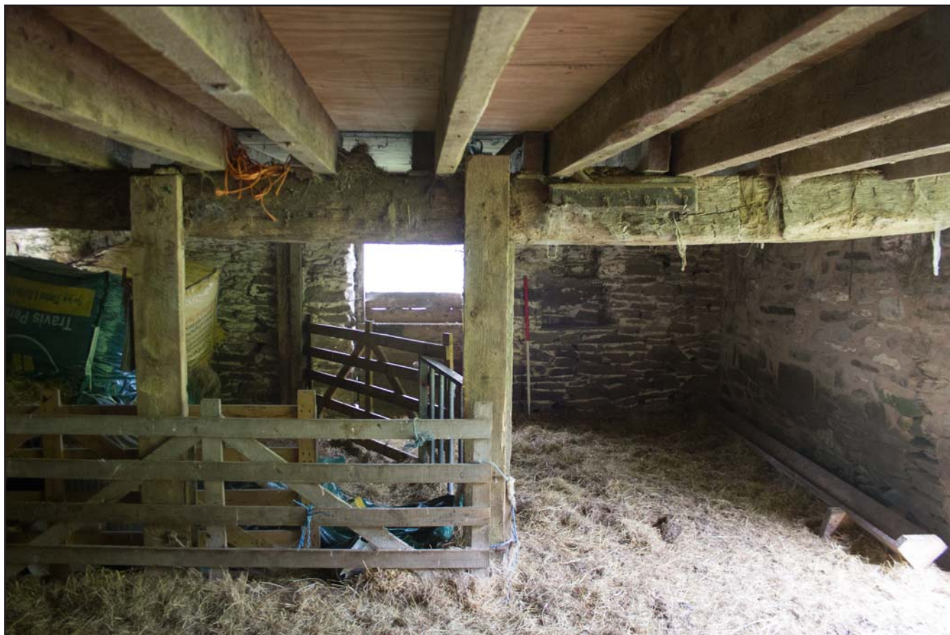
Plate 08: Ground floor barn at Hen Hafod, Nantyr, from the southwest. Scale 1.0m.
