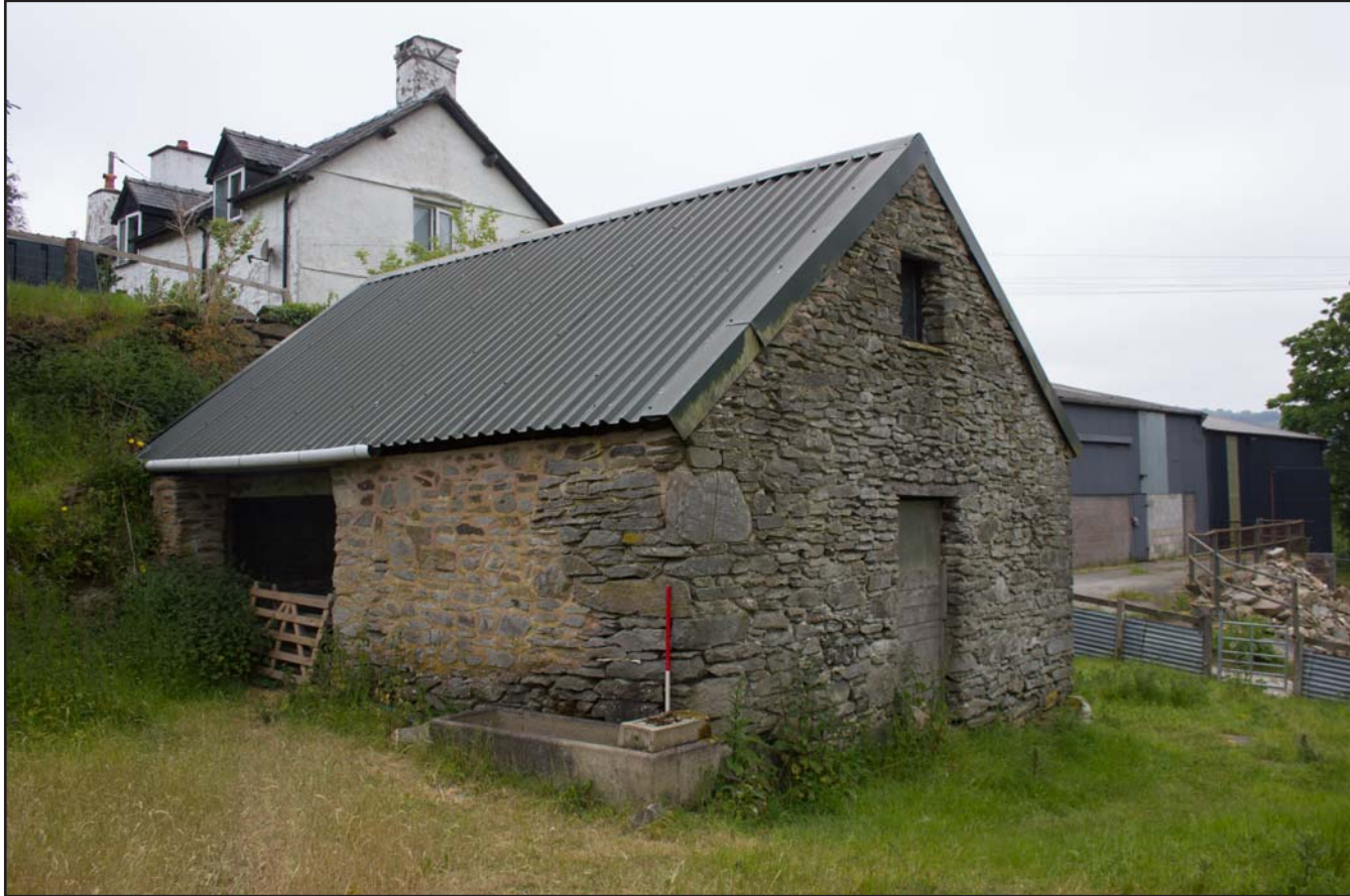
Plate 05: Northeast and southeast facing external elevations of barn at Hen Hafod, Nantyr, from the east. Scale 1.0m.
