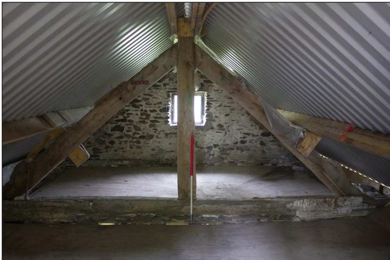
Plate 13: First floor hay loft at Hen Hafod, Nantyr showing king-post truss, from the southwest. Scale 1.0m.
