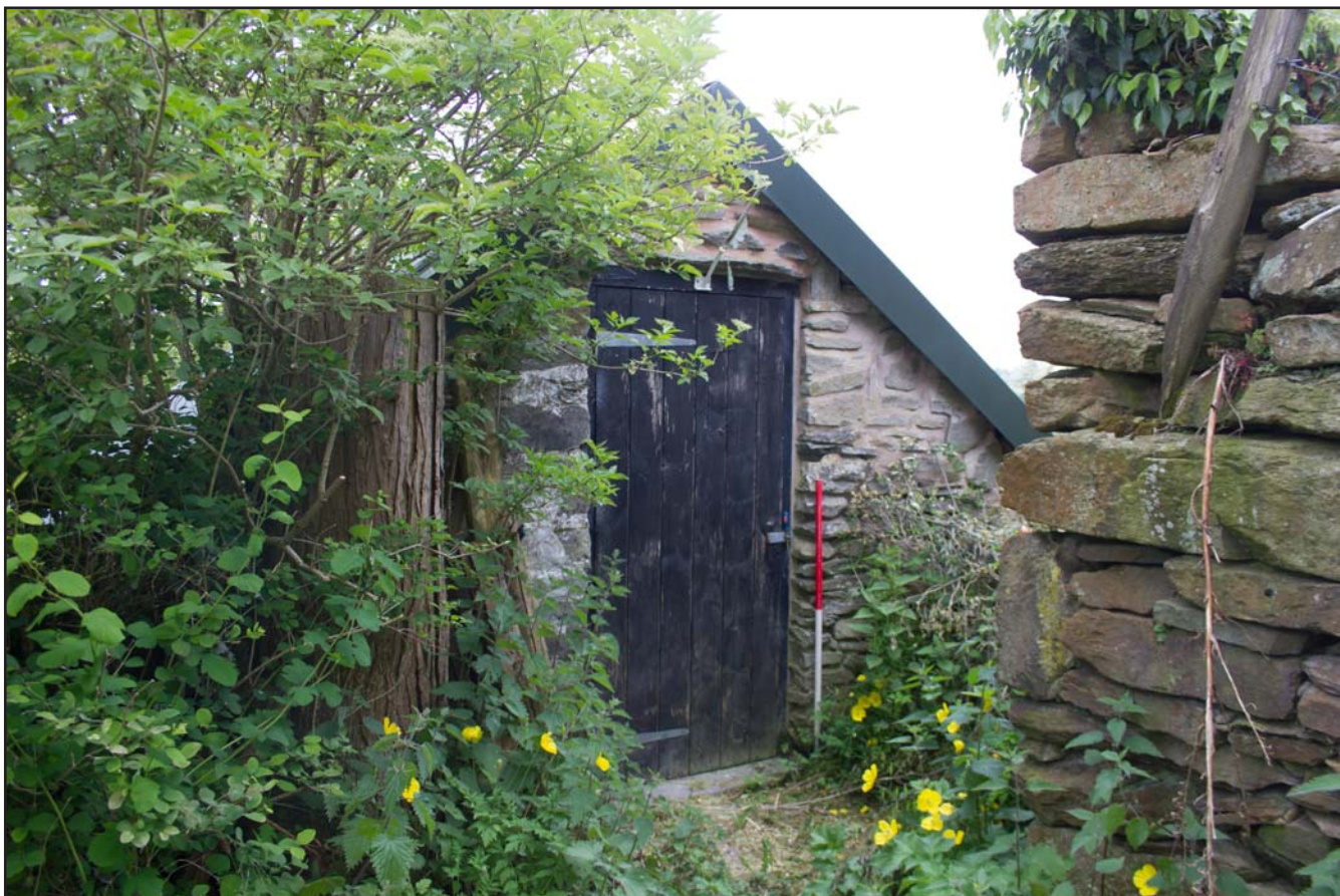
Plate 07: Southwest facing external elevation of barn at Hen Hafod, Nantyr, from the west. Scale 1.0m.
