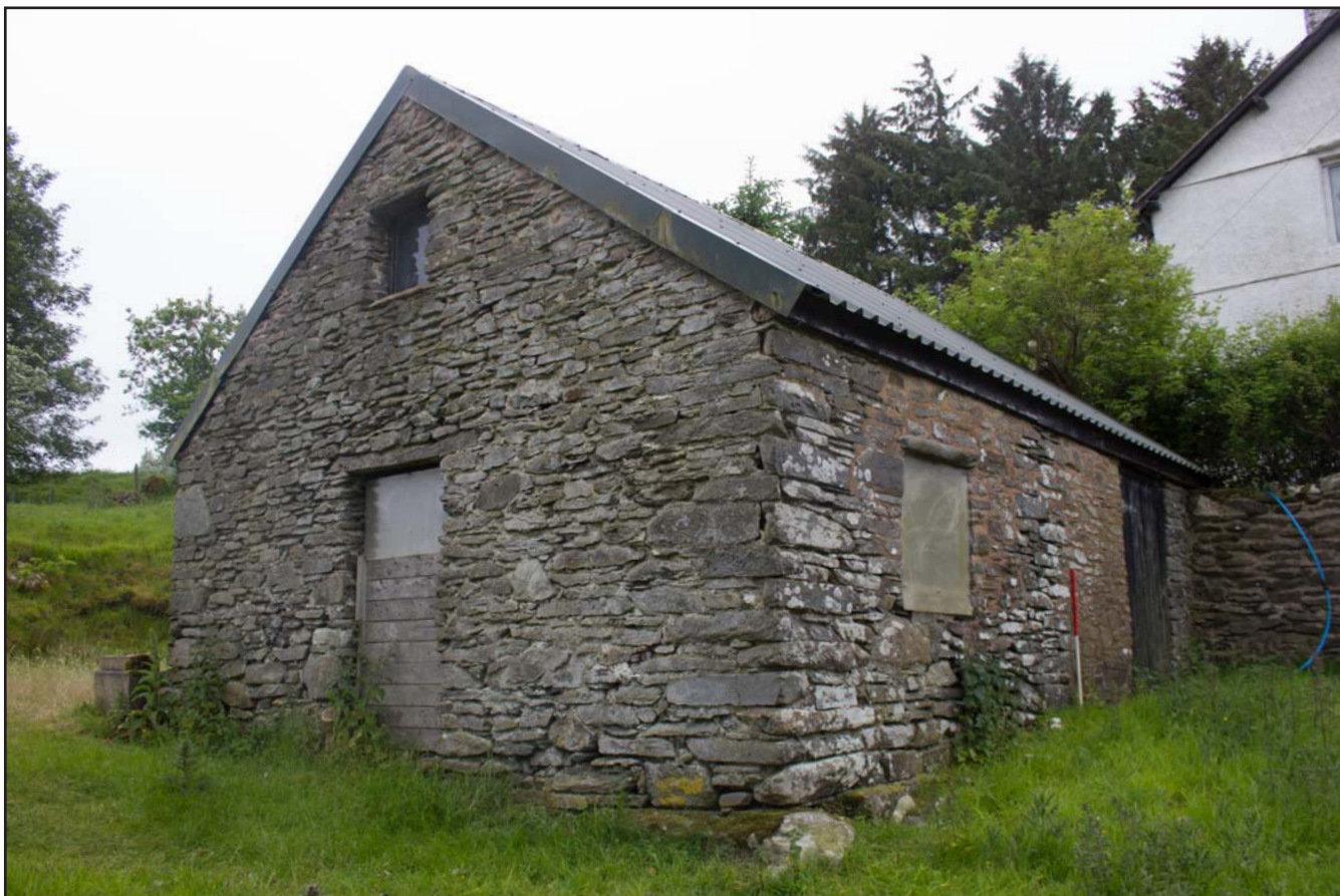
Plate 03: Northwest and northeast facing external elevations of barn at Hen Hafod, Nantyr, from the north. Scale 1.0m.
