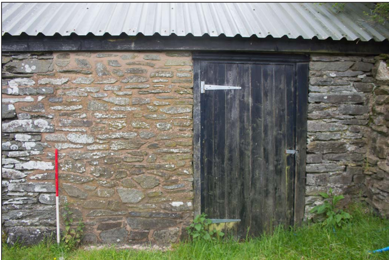
Plate 02: Northwest facing external elevation of barn at Hen Hafod, Nantyr showing rebuilt masonry, from the northwest. Scale 1.0m.
