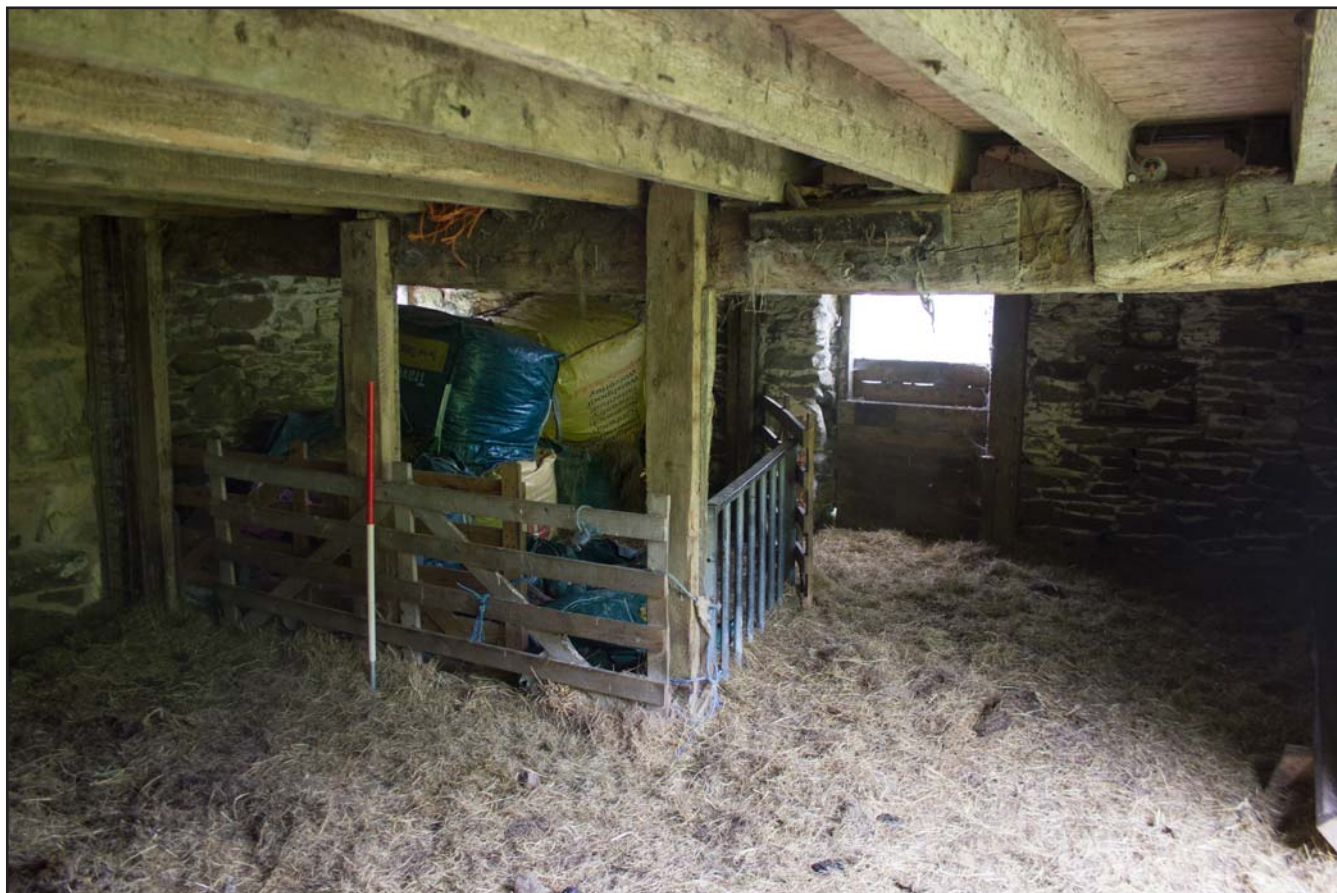
Plate 09: Ground floor barn at Hen Hafod, Nantyr, from the south. Scale 1.0m.
