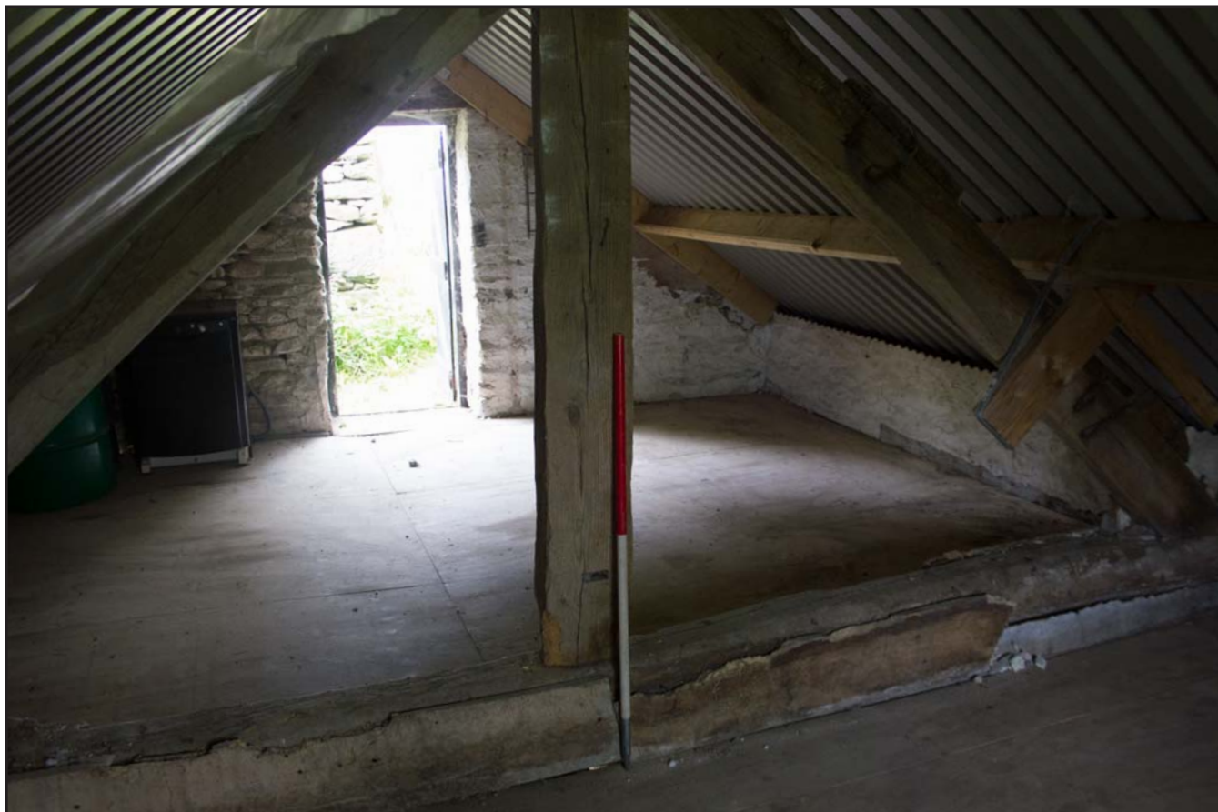
Plate 14: First floor hay loft at Hen Hafod, Nantyr showing king-post truss, from the east. Scale 1.0m.
