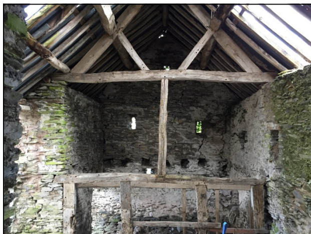
Plate 1 Looking east through pitched roof section of barn
