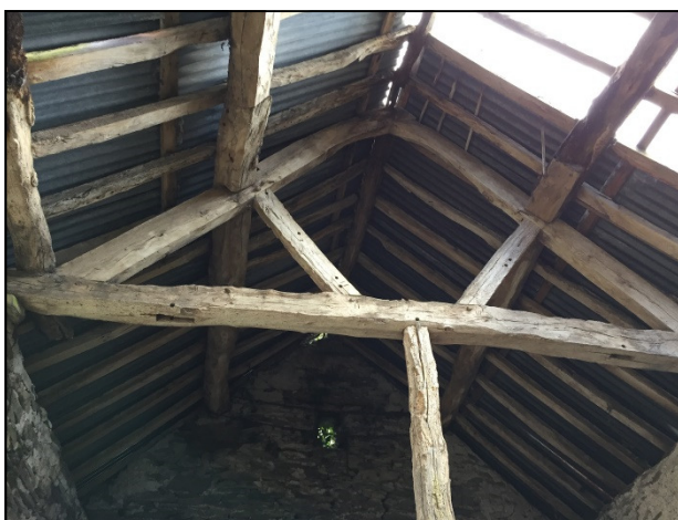
Plate 4 Roof timbers support mortise and tenon joints
