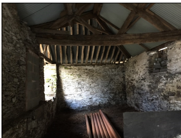
Plate 2 Looking south through hipped roof section of barn
