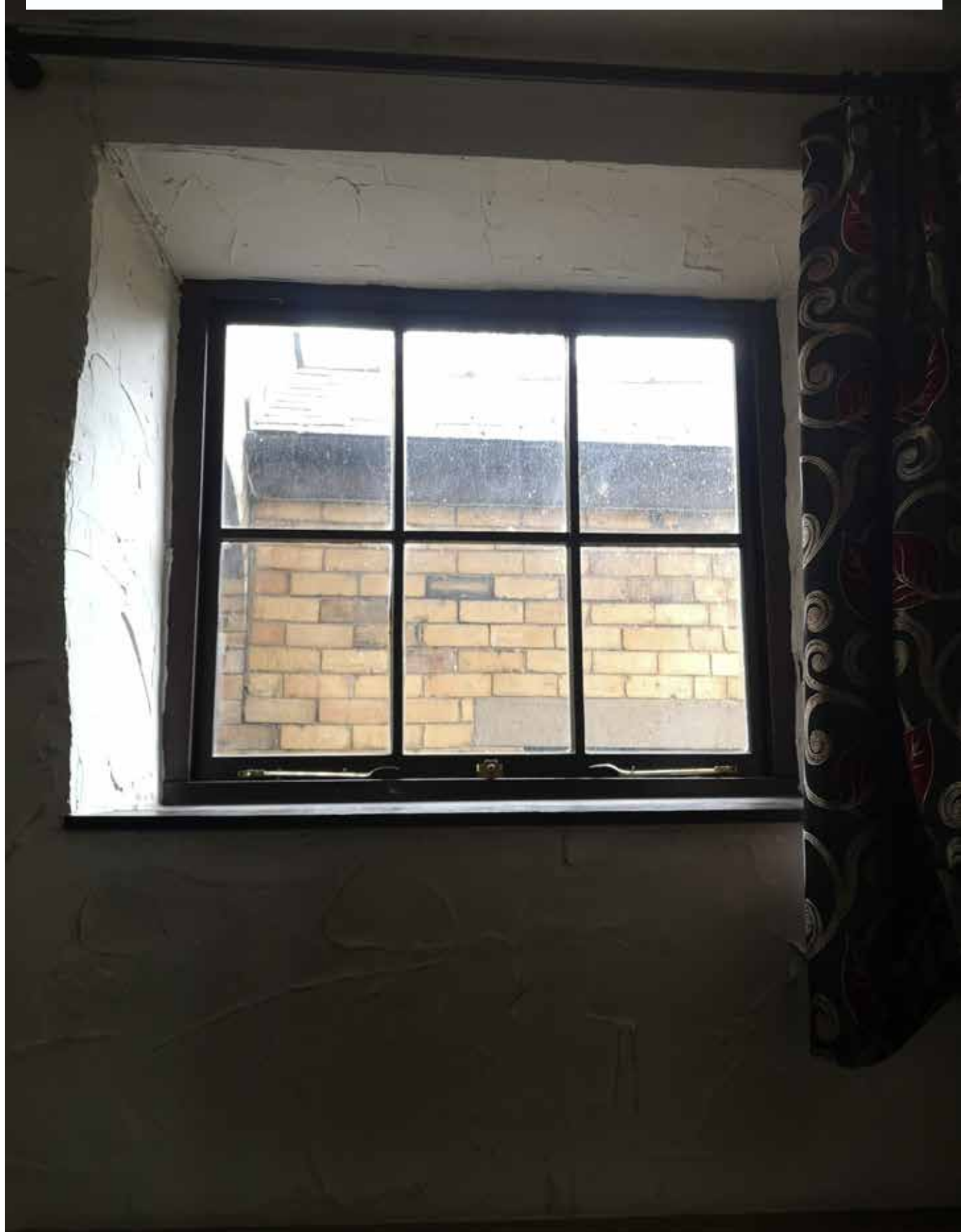
East elevation interior view of ground floor lounge window.
