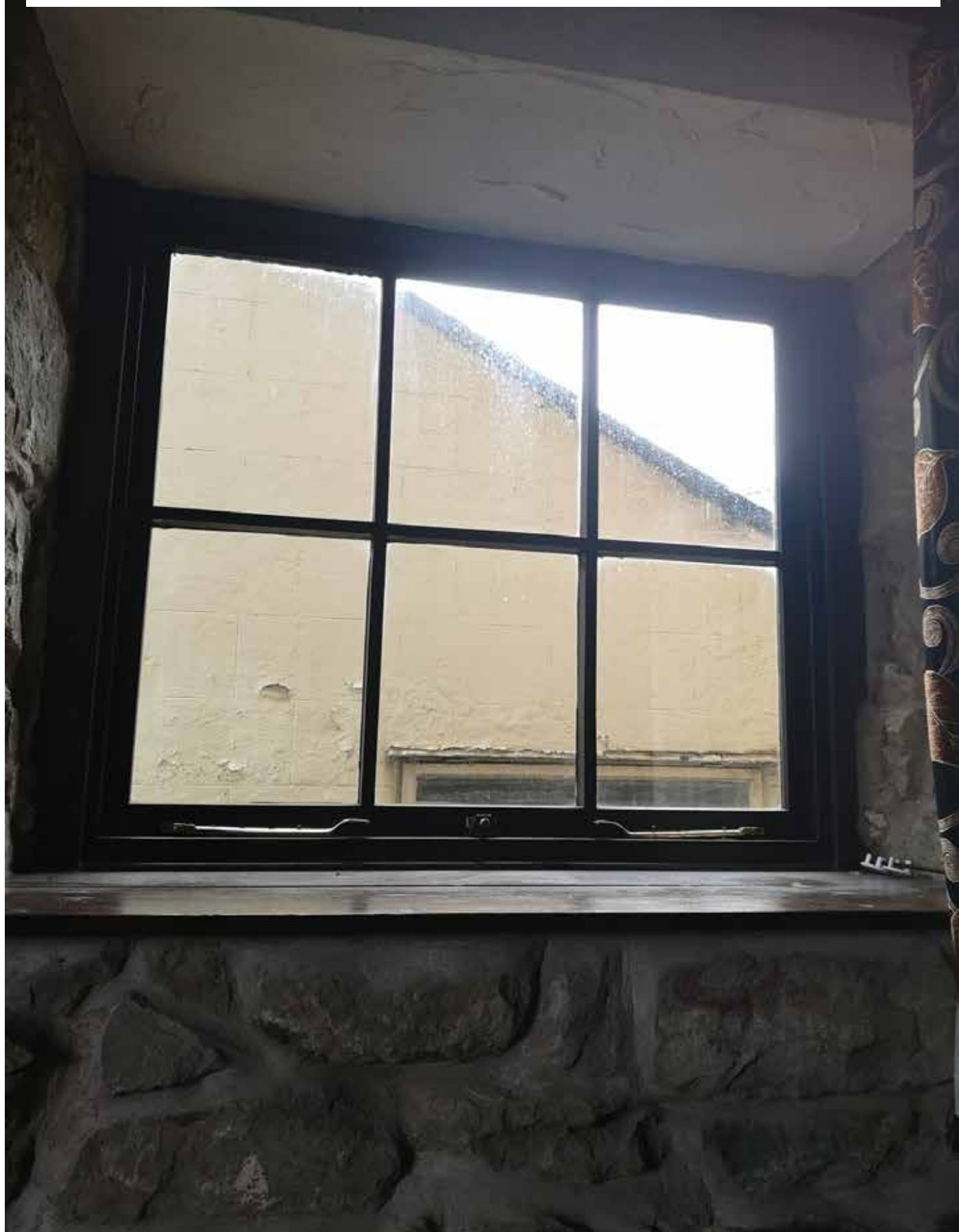
West elevation interior view of ground floor lounge window.
