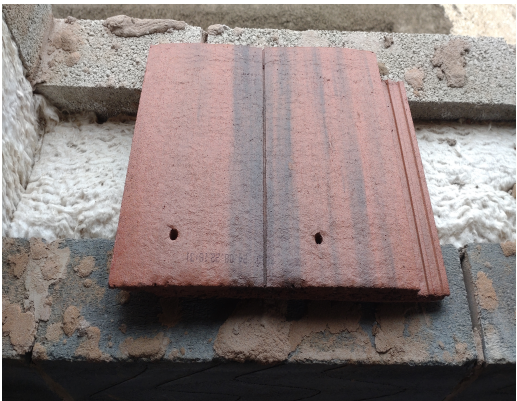
Marley Ashmore Old English Dark Red tiles installed to garage and dwelling roof altereing previously approved roof tile.
