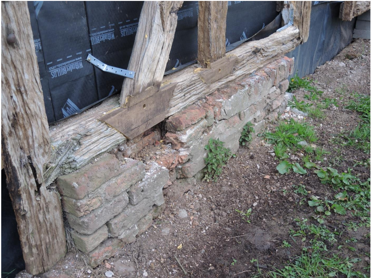
Figure 14 – Shippon 1: Existing brick plinth and the adjacent 'pitched' cobbled yard surface to the NE elevation
