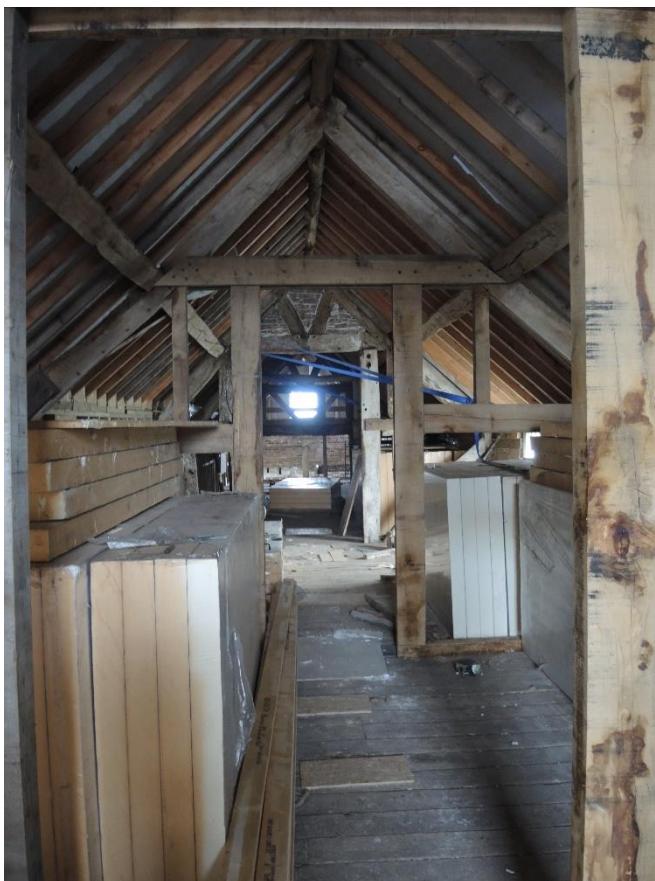
Figure 18 - Shippon 1 First Floor image towards the NW gable
