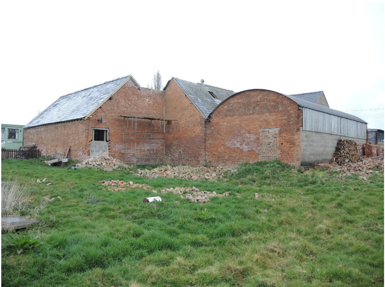
Figure 11 - Shippens 2, 3 and Building 04: Existing SW and NW elevations
