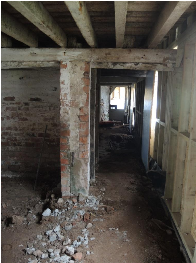
Figure 16 + 17 - Shippon 1: Ground floor image of the floor, the timer lining and the existing first floor joists and boards
