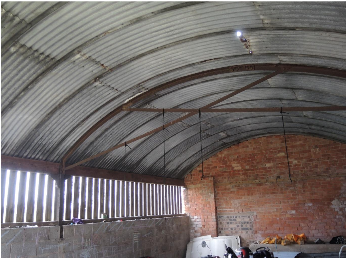
Figure 21 - Building 4 - Existing corrugated metal roof covering and structure, together with the SE + SW facing walls
