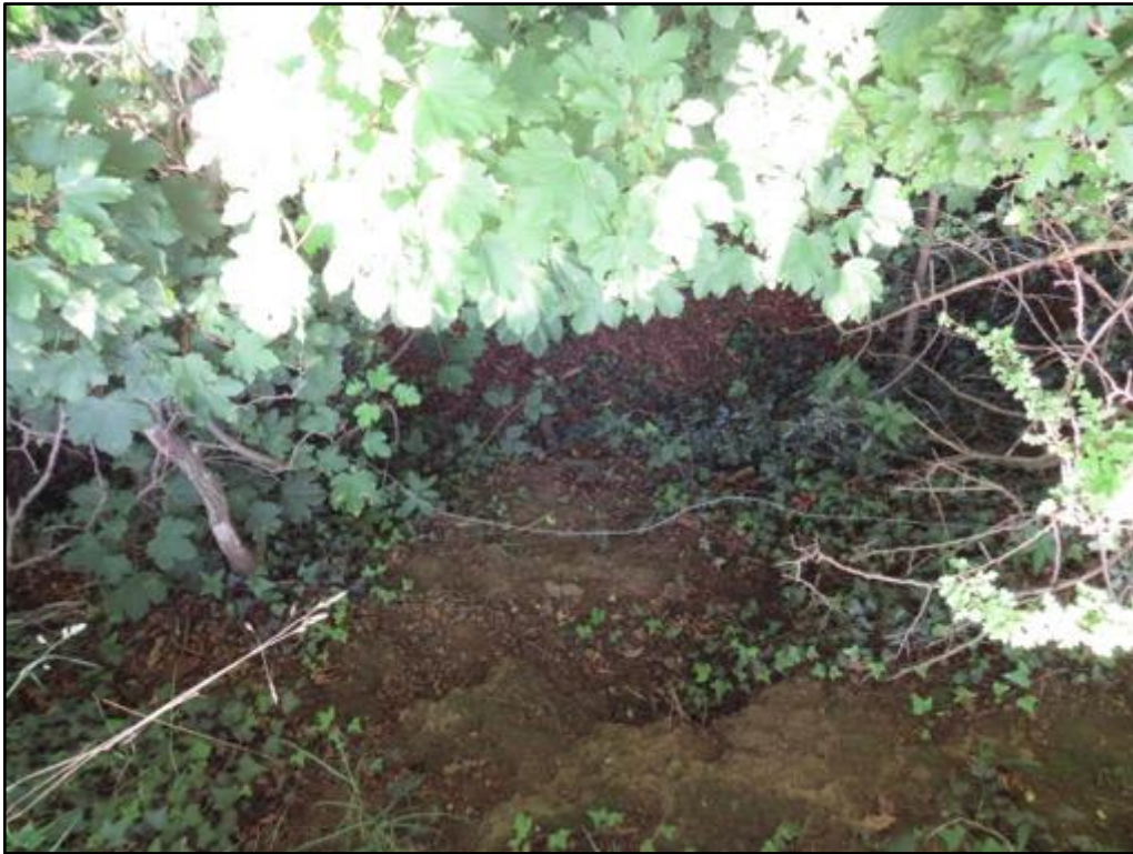
Photograph 13: A drain runs within the eastern hedge boundary; this is in a dry state.
