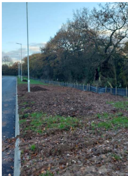
Heras fencing removed and duct backfilled.
