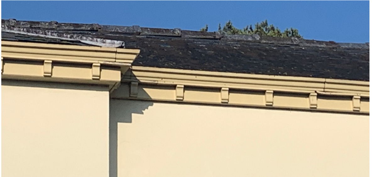
Photograph 3. Example damage to soffit boxes
