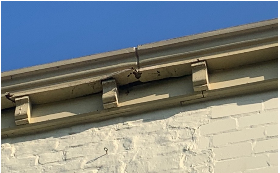
Photograph 3. Example damage to soffit boxes
