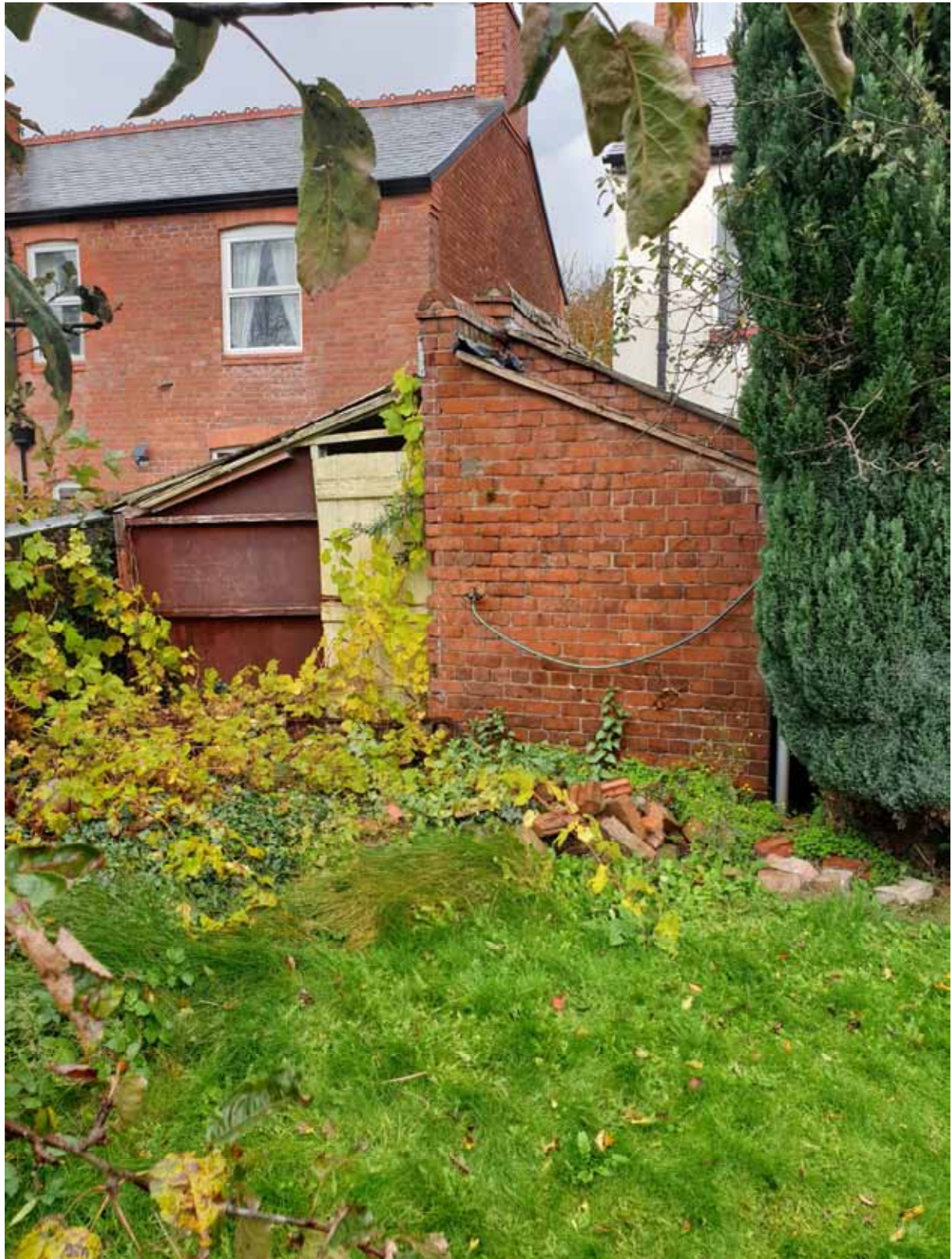
Rear Elevation of Outbuilding & Garage:
