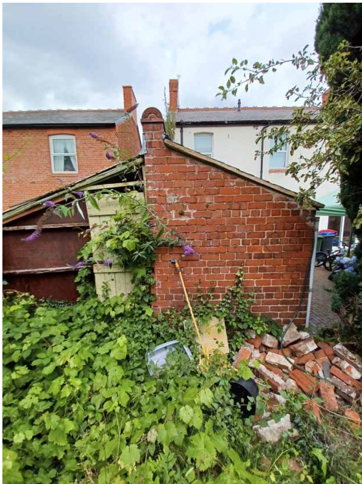
Rear Elevation of Outbuilding & Garage:
