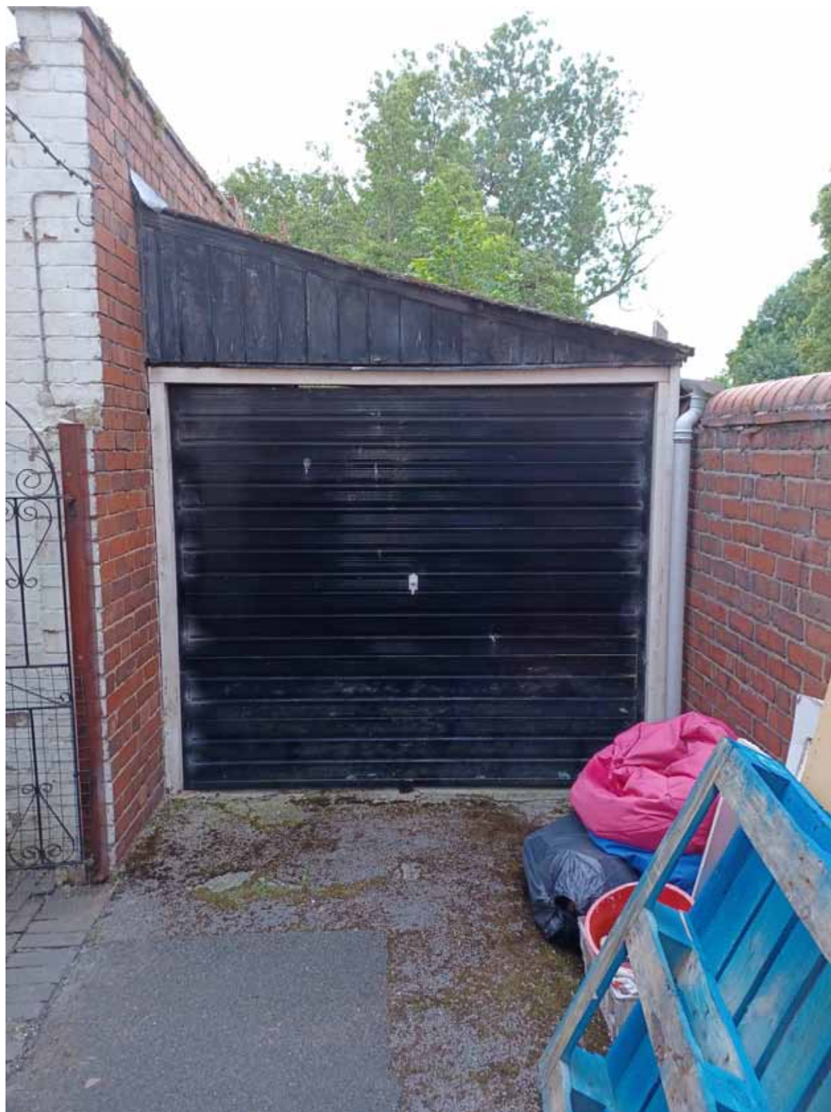
Front View Of Garage Abutting Outbuilding And Boundary Wall:
