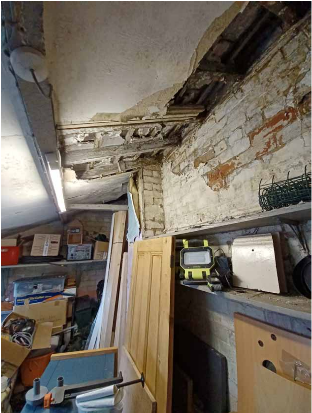
Chimney Breast At High Level:
