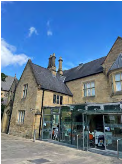
Photograph 1 – Northern aspect of building, looking to east.
