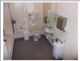
Photo WCM20 - Accessible toilet first floor
