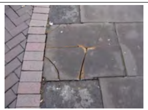
Photo WCM03 - side car park paving
