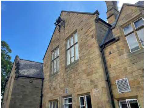
Photograph 4 – western aspect of building showing gable ends
