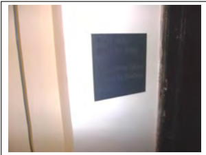
Photo WCM18 - Signage on first floor
