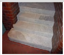
Photo BLM23 - Side stairs to first floor
