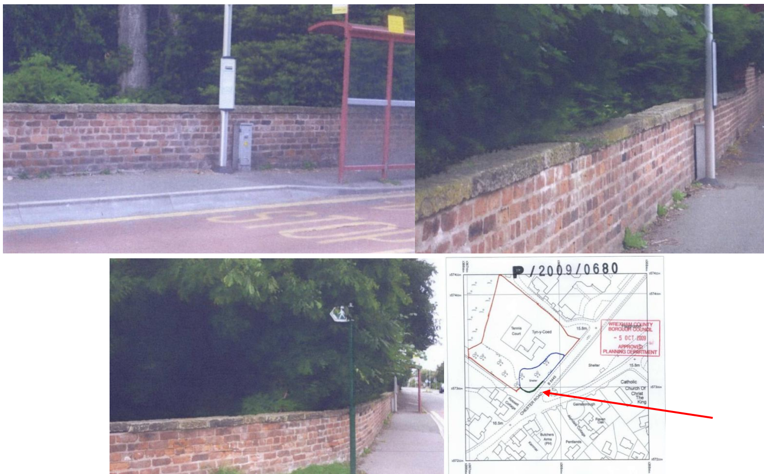
Fig 6. Planning application photographs of 2009 showing the wall had been reduced in height since the 1960's, and permission granted in 2009 to rebuilt up at the corner (arrowed red).
