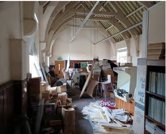
A high significance space that is currently under-utilised and filled with storage
