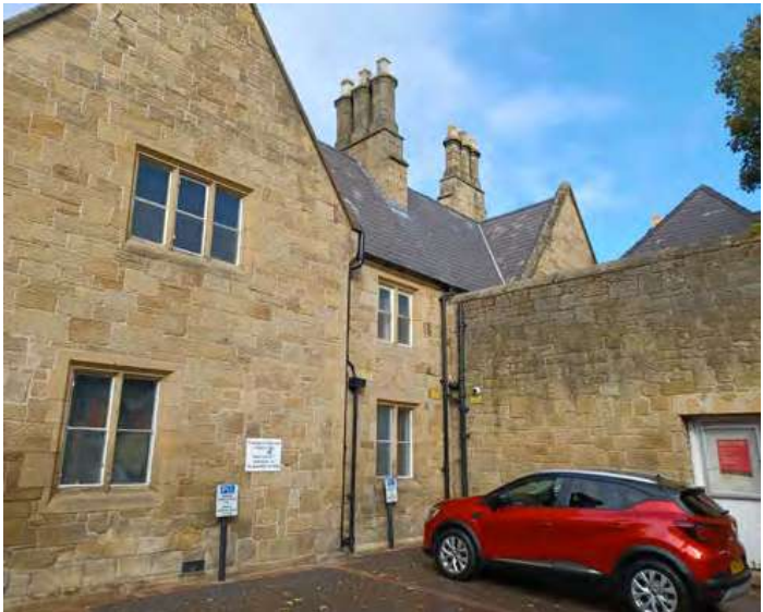
The disabled parking spaces to the side of the building
