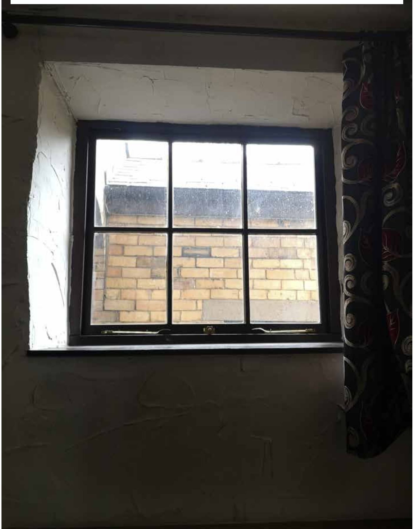
East elevation interior view of ground floor window.
