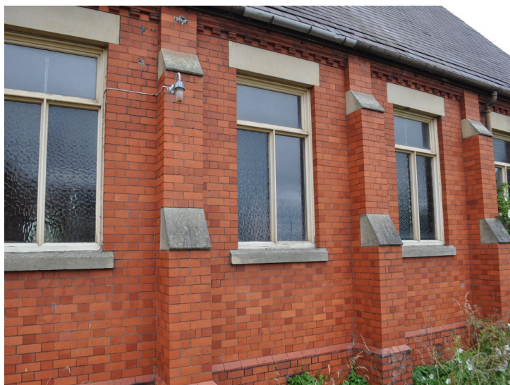
Plate 15 - East elevation, detail
