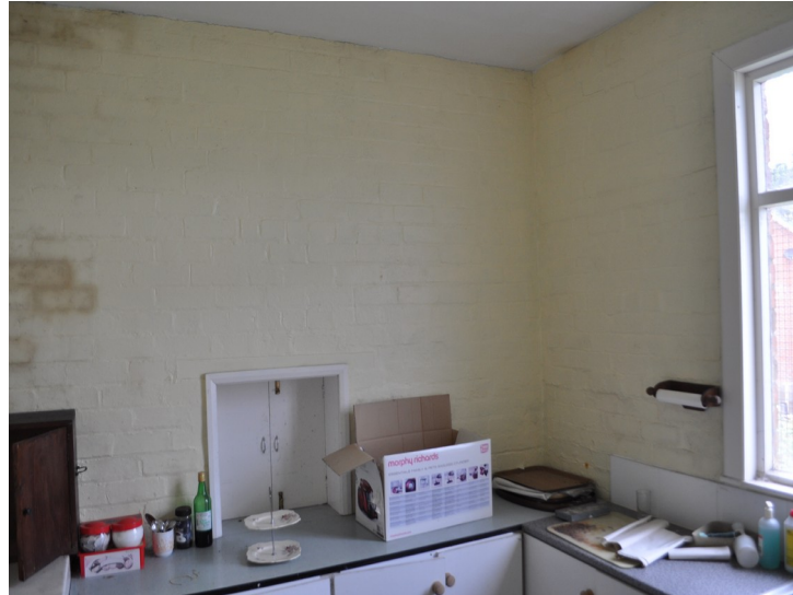
Plate 36 - Kitchen, looking west
