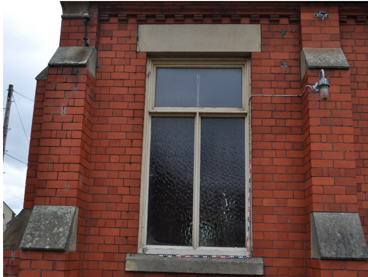
Plate 16 - East elevation, southernmost window detail
