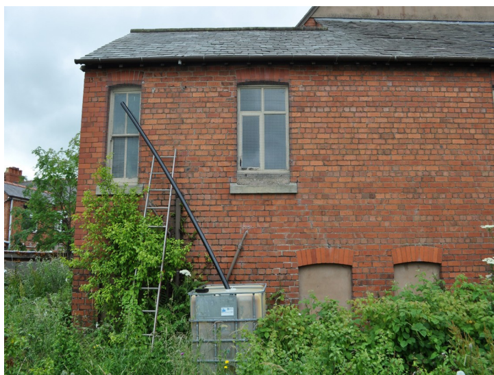
Plate 21 - North elevation of vestry
