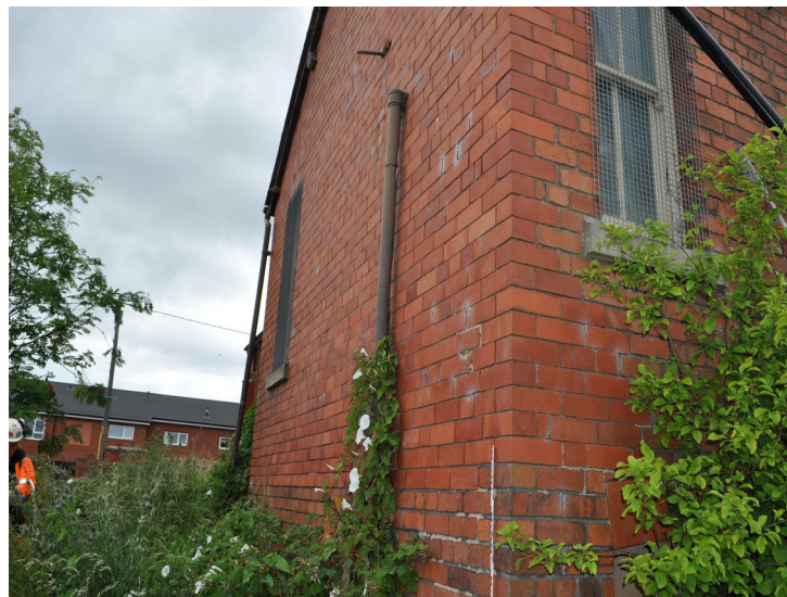
Plate 18 - East elevation of vestry
