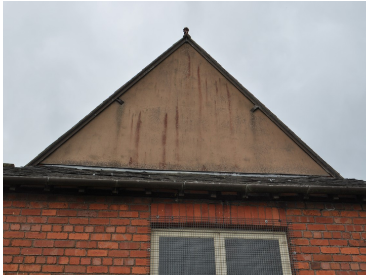
Plate 19 - North elevation, rendered wall and finial
