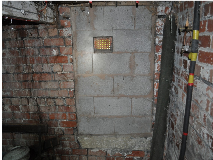
Plate 45 - Breeze blocked window on north wall of cellar
