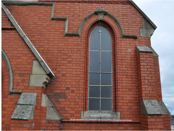
Plate 8 - South elevation, east window
