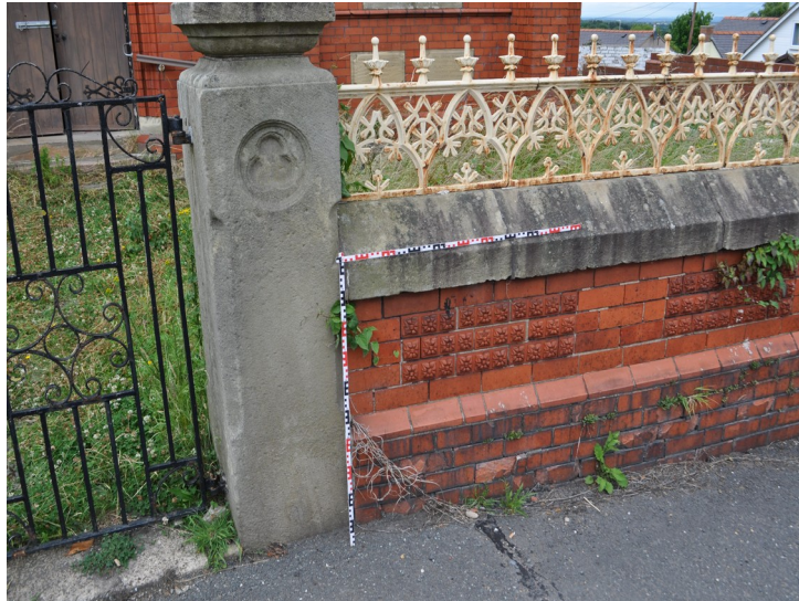
Plate 4 - Exterior wall, panel and fence detail
