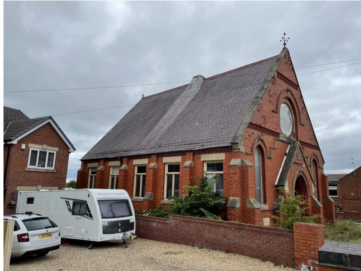
Plate 1 - View of Salem Chapel, looking northeast
