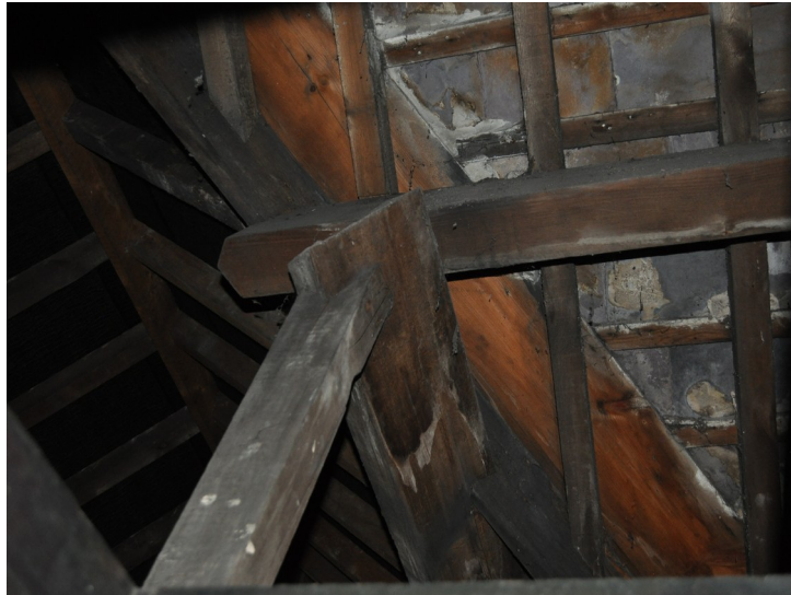
Plate 41 - Roof structure in annex
