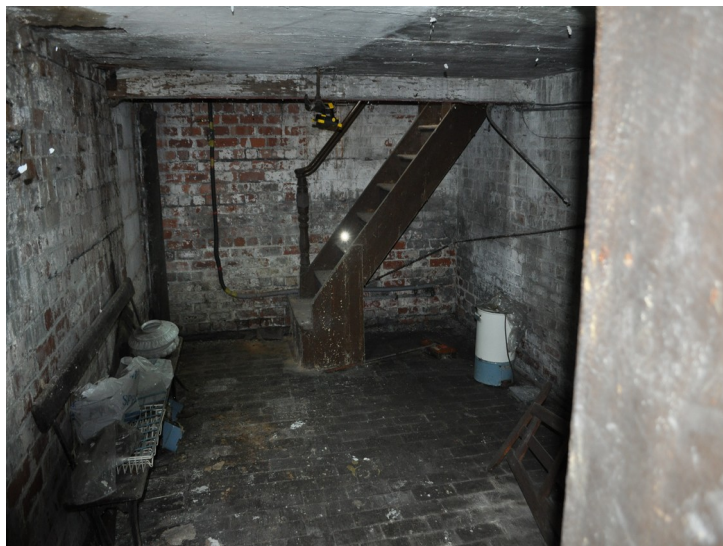
Plate 42 - Access to cellar, looking east
