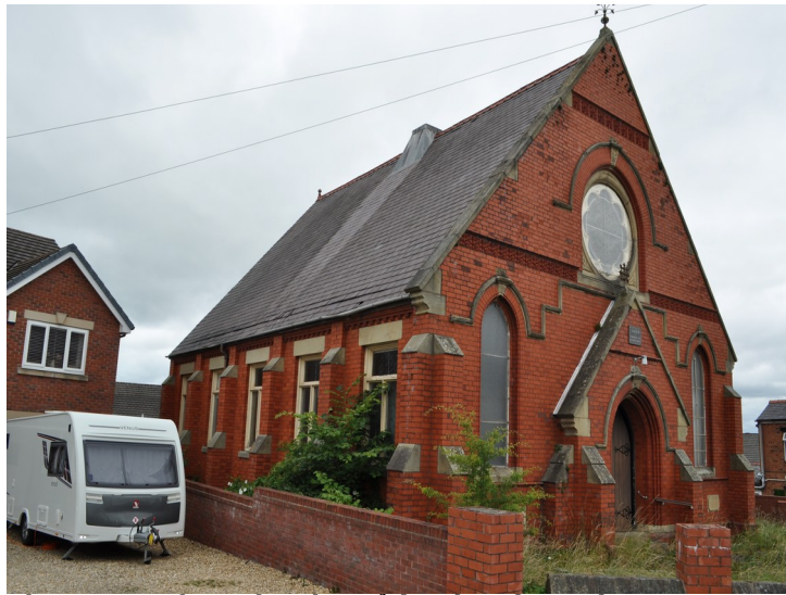
Plate 24 - Salem Chapel, roof detail with weathervane, zinc chimney and finial (Right to left)
