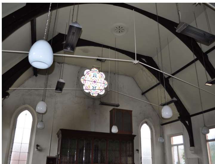
Plate 32 - Hammer beams, tie-beams, ceiling vents and lighting detail
