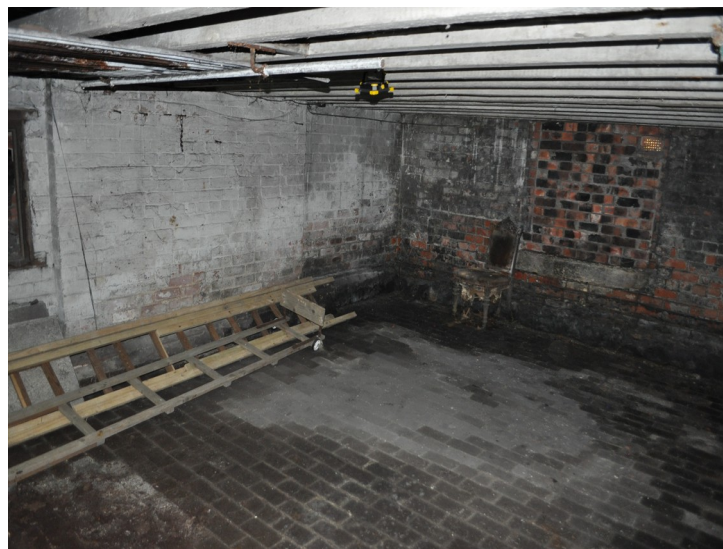
Plate 46 - Main cellar room
