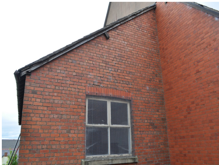
Plate 23 - West elevation of vestry, with window
