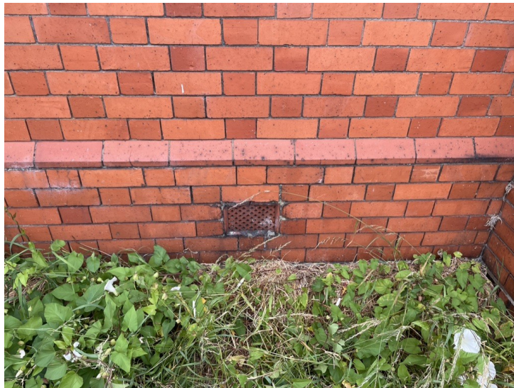
Plate 17 - Base of eastern elevation
