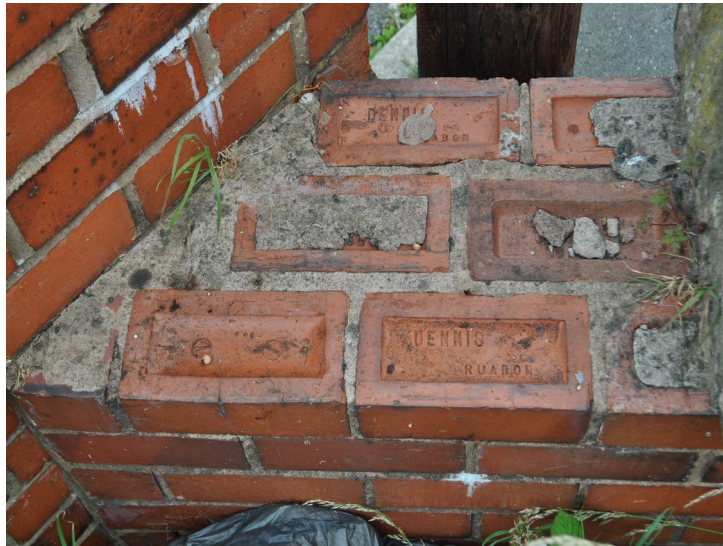
Plate 3 - Exterior wall, brick detail
