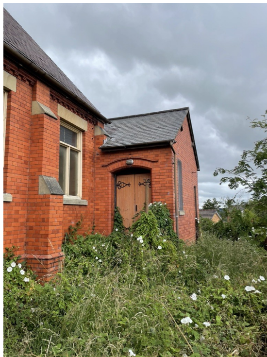
Plate 12 - Vestry, looking north
