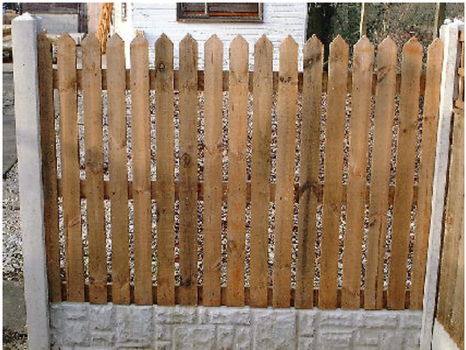
Palisade fence panels above gabions (Rear boundary only)
