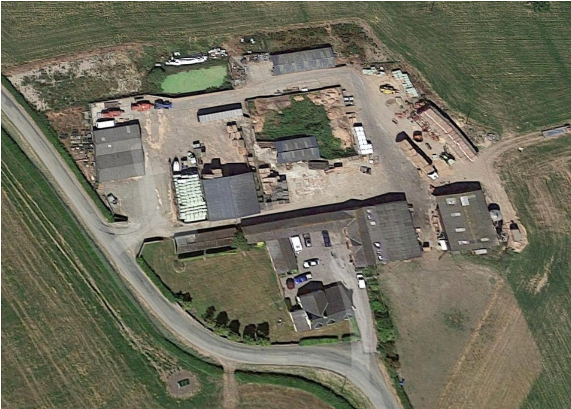
Aerial Image of Mulsford Farm
