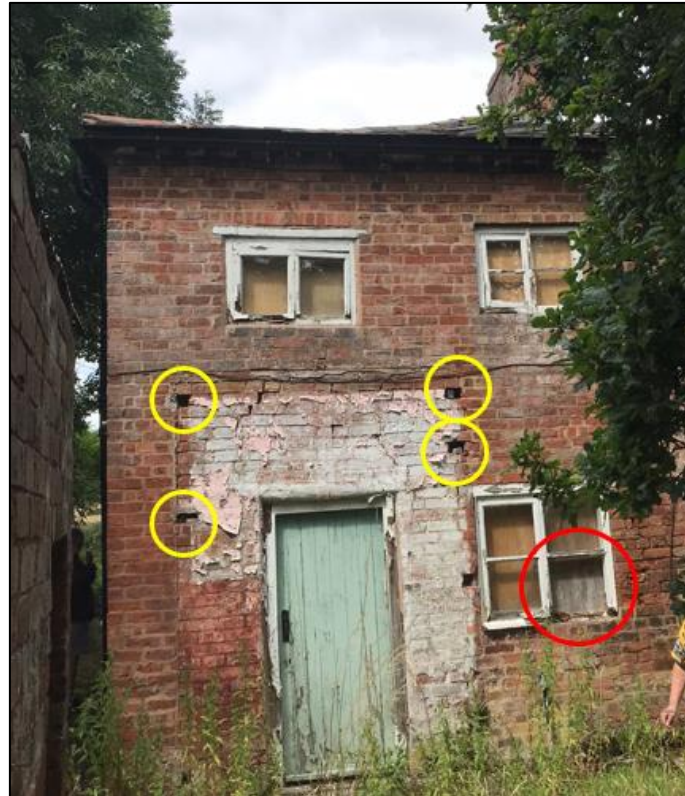
Plate 10. Gap above the front door
