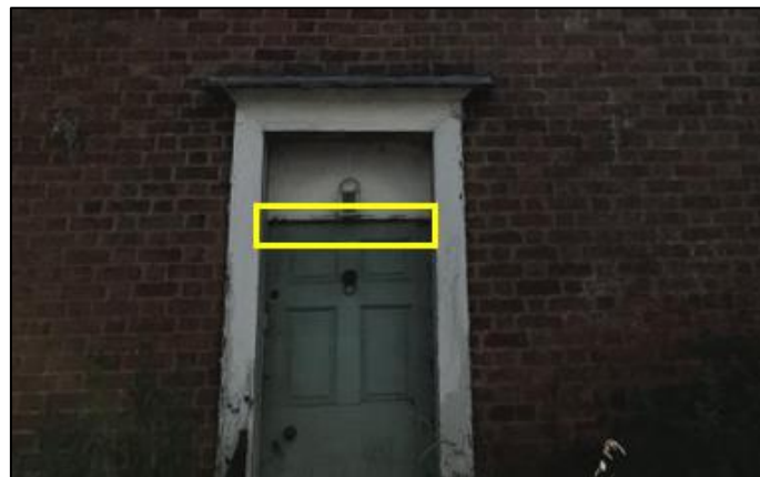
Plate 10. Gap above the front door
