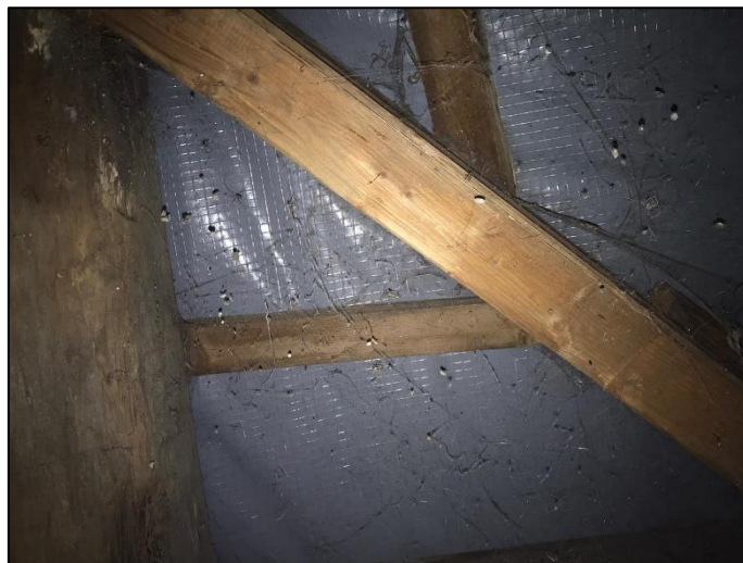
Plate 8. Loft roof beams and roof membrane
