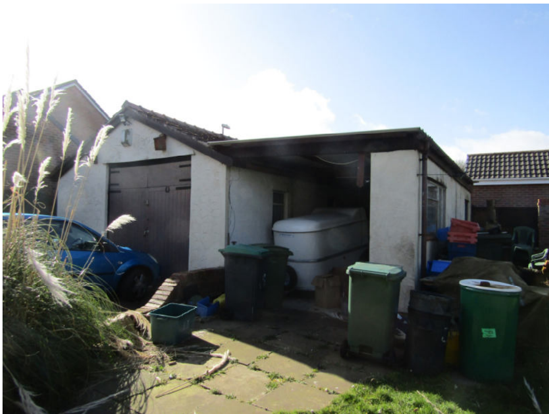
Photo 4: Garage [J3.6] was assessed as having low potential for roosting bats.
